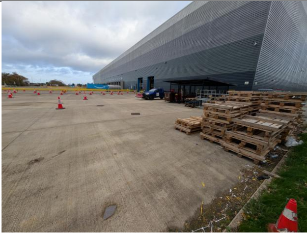
Photograph 1 – The south side of the warehouse which shows the hardstanding where the proposed location for the air source heat pumps and elevation alterations to include new louvres is.
