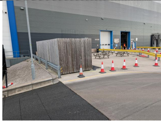
Photograph 2 - The south side of the warehouse which shows the hardstanding where the proposed location for the refrigeration plant enclosure is.
