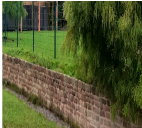
Photograph 14: Stone wall and mesh fencing in the south standing east facing west
