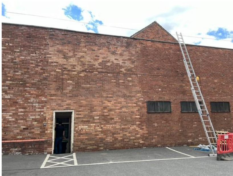
Wall to the rear of the building
