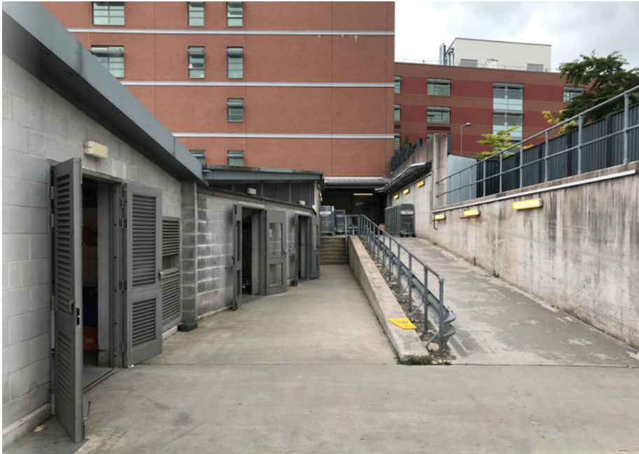
Existing operations - bin stores, ramp, retaining wall
