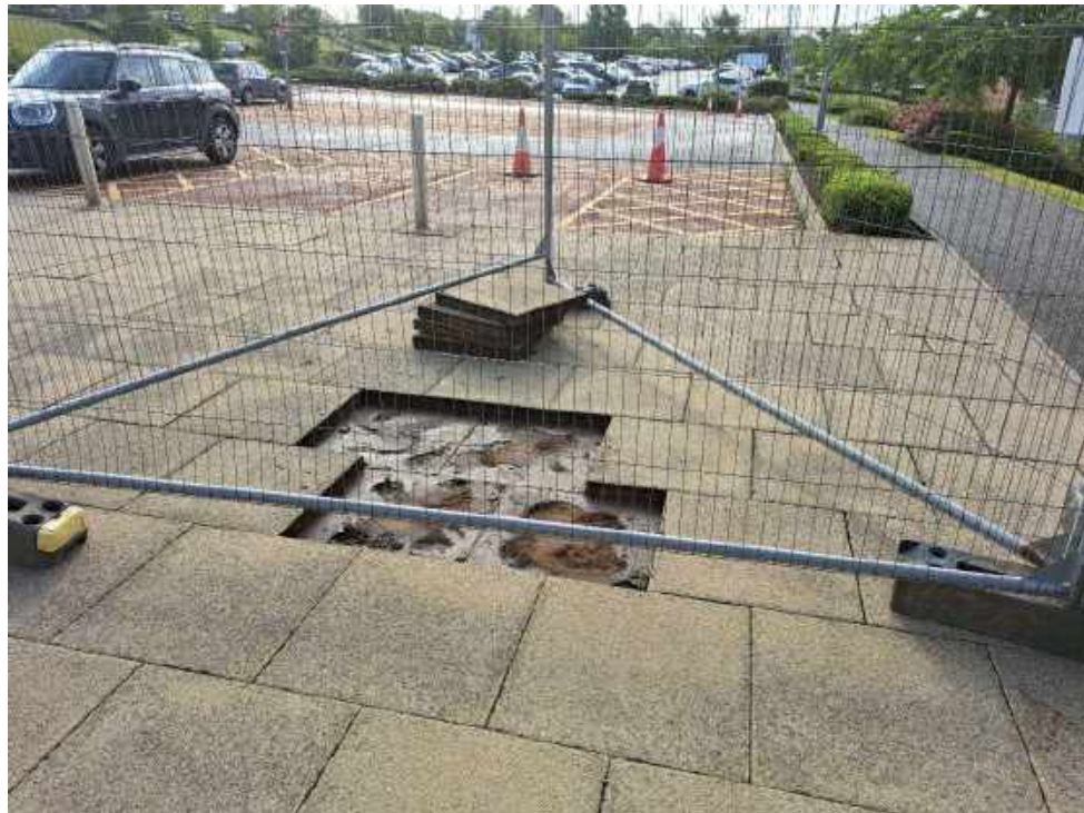
Photograph 13 BH01 at start of works
