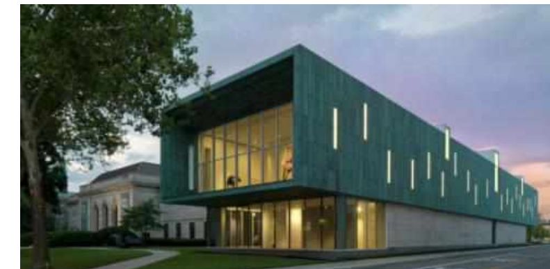
Metal cladding to upper floors with picture windows at the end.
