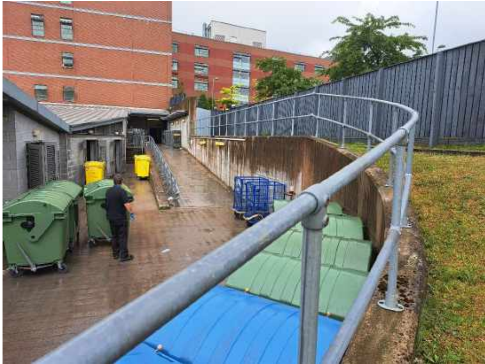
Photograph 3 Retaining wall, bin store and ramp in south of site
