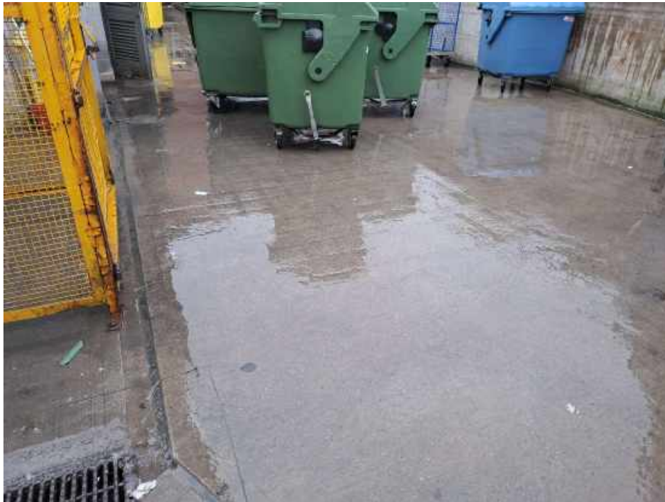
Photograph 1 Concrete hardstanding at base of retaining wall / ramp in southern area of site
