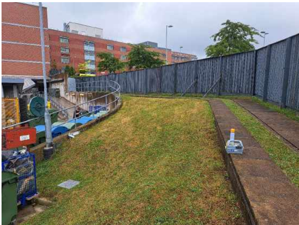
Photograph 2 View north-east across site. Retaining wall and ramp visible in left of image, covered utility ducting visible to right of image, and steep grassed slope in centre of image.
