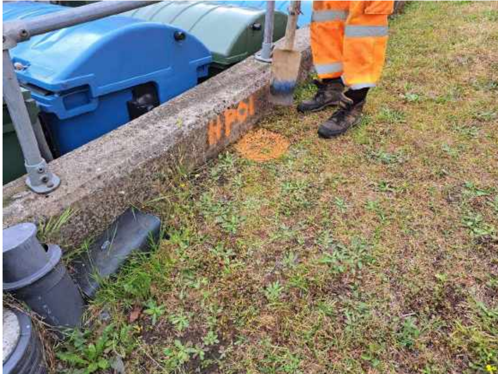
Photograph 10 Hand pit HP01 prior to start of excavation
