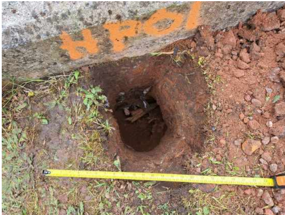
Photograph 11 Hand pit HP01 open excavation showing vertical geotextile membrane on far edge of hole and horizontal geotextile at depth
