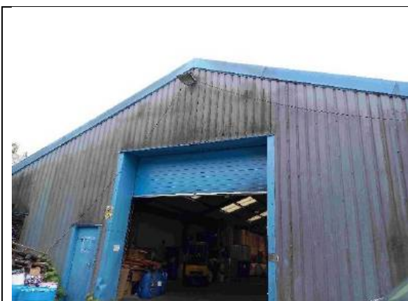
Photograph 17: Western elevation of B3
