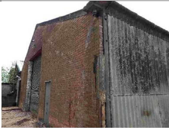
Photograph 13: Eastern and northern elevation of building B2
