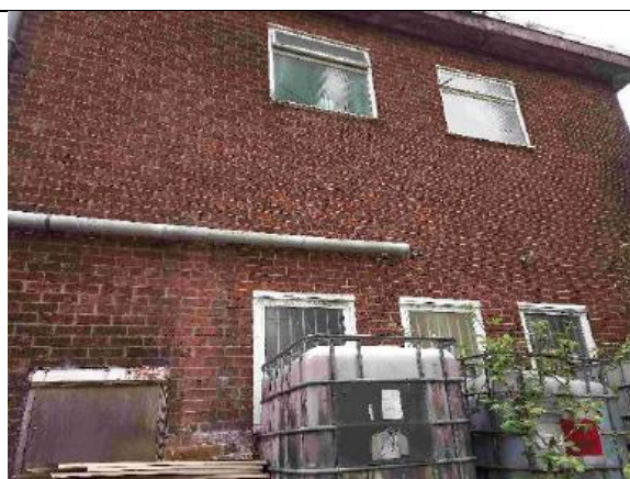
Photograph 20: Eastern elevation of B4
