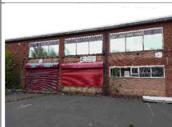
Photograph 19: Southern elevation of B4
