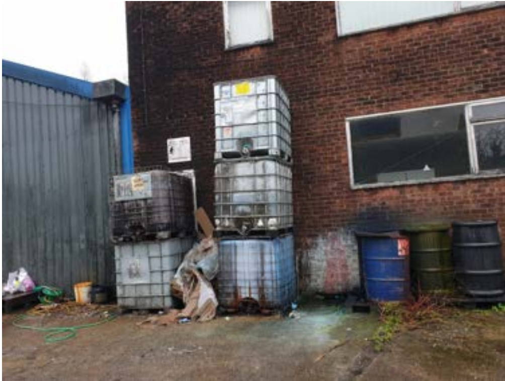
Photo 49: View of IBC's and chemical drum storage outside buildings and associated spillage on concrete floor (looking E).
