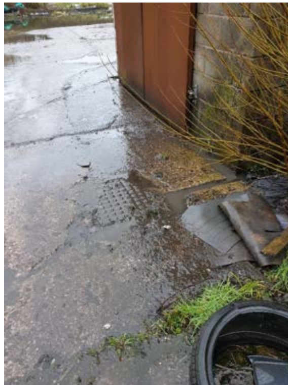
Photo 54: View of manhole next to roofed storage area in N of site.
