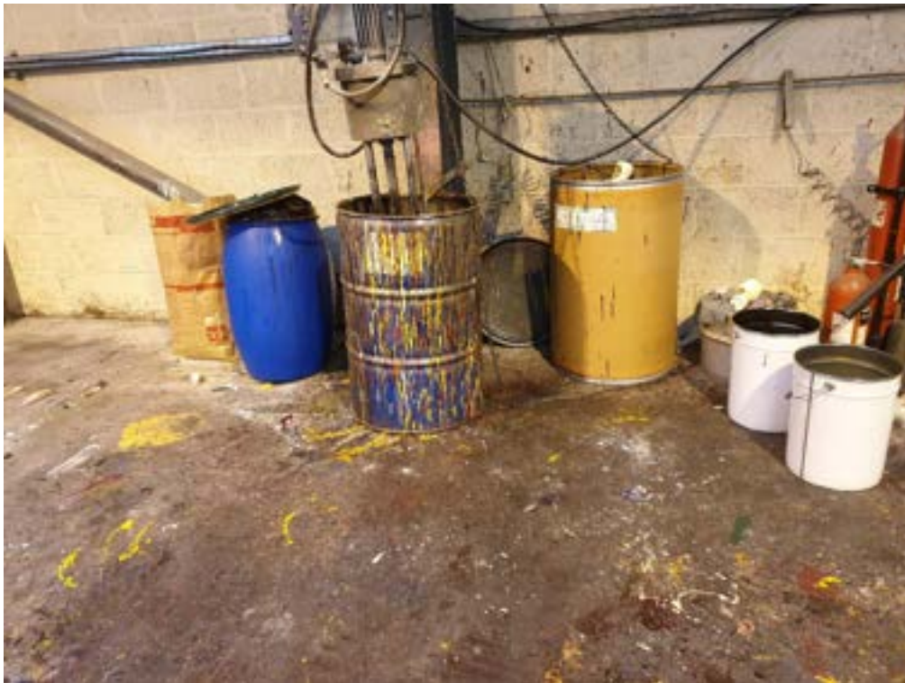
Photo 9: Northern wall of inside the middle building, showing chemical storage drums and noticeable spillages on the floor.
