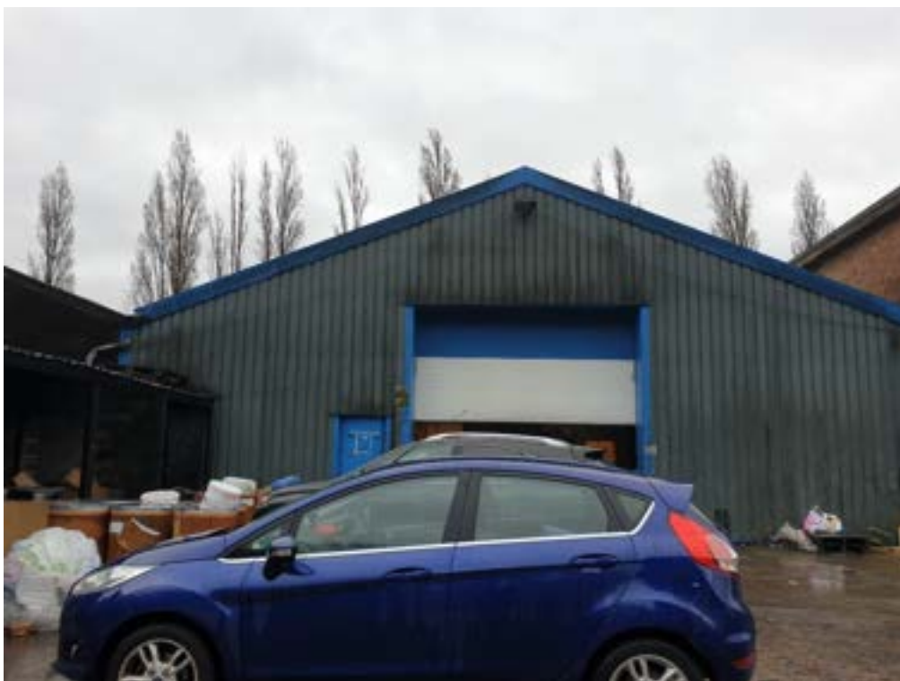
Photo 6: View of middle building, looking to the east of the site.
