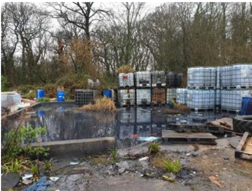
Photo 30: Bunded area in NW of site (looking across west boundary) showing polluted surface water and IBC's.
