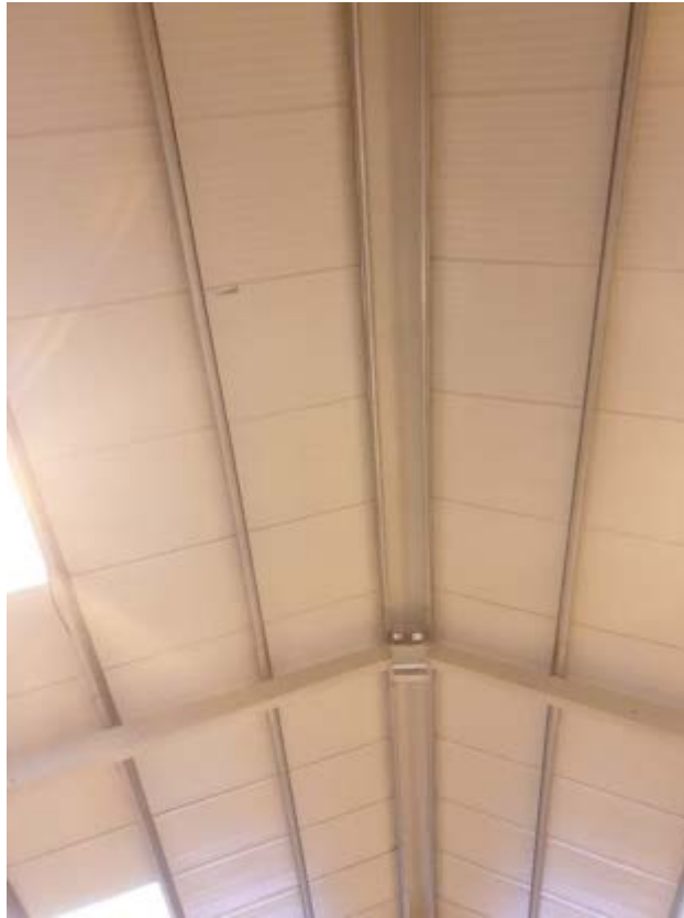
Photo 7: View of internal roof of the middle building.
