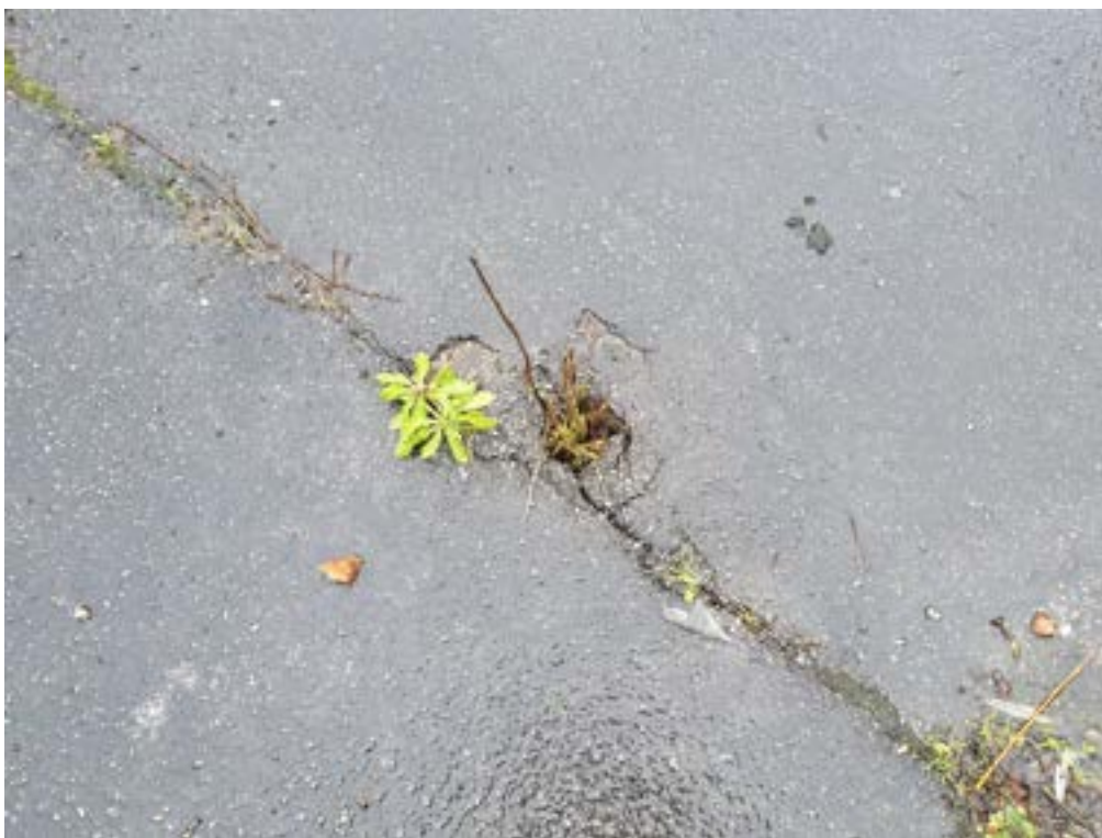
Photo 22: View of potential borehole from prior Phase 2 and 3 investigations (taken in SE of site).
