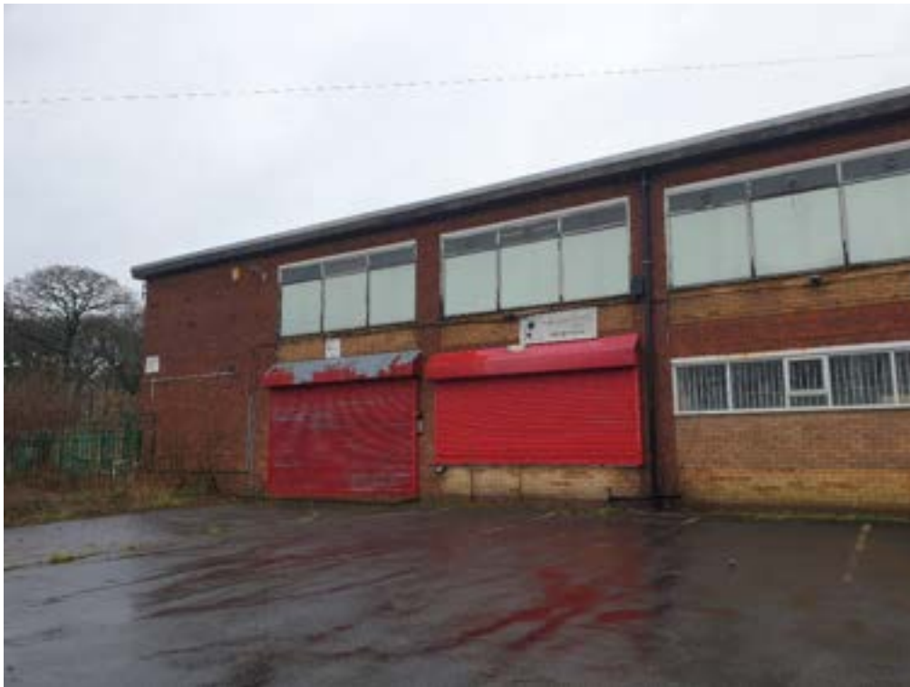
Photo 19: View of most south building and tarmac area to the south of it (taken from SE looking N).
