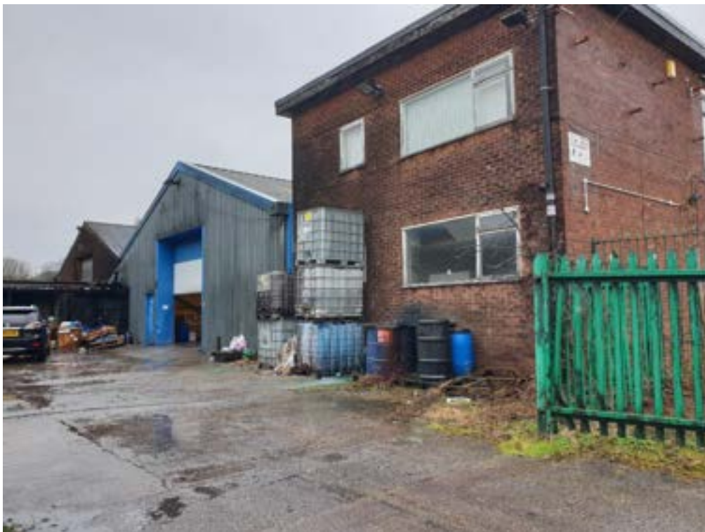
Photo 2: View of three adjoining buildings, from the centre of the site looking NE.
