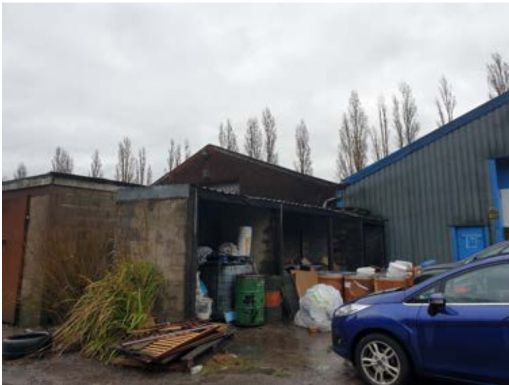
Photo 4: View of open, roofed storage area (looking NE) showing the middle and most northern building in the background.
