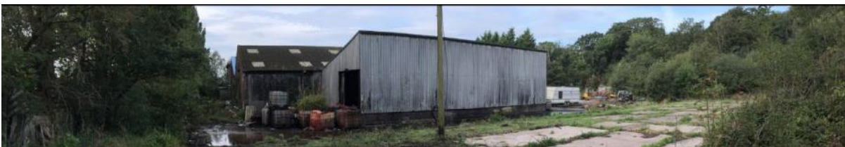
Figure 1 – Photos of the existing buildings at the application site.
