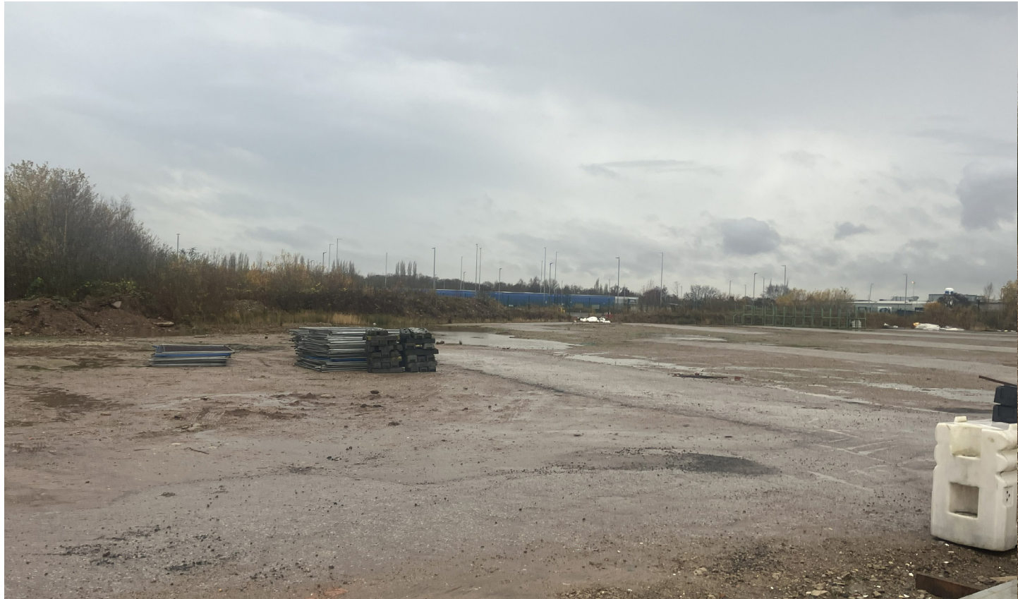
Image 1-3. Existing carpark hardstanding
