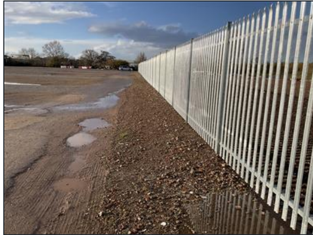
Photograph 5 – Urban built linear feature, (fence). Located sectioning off the northern unsealed surface habitat.
