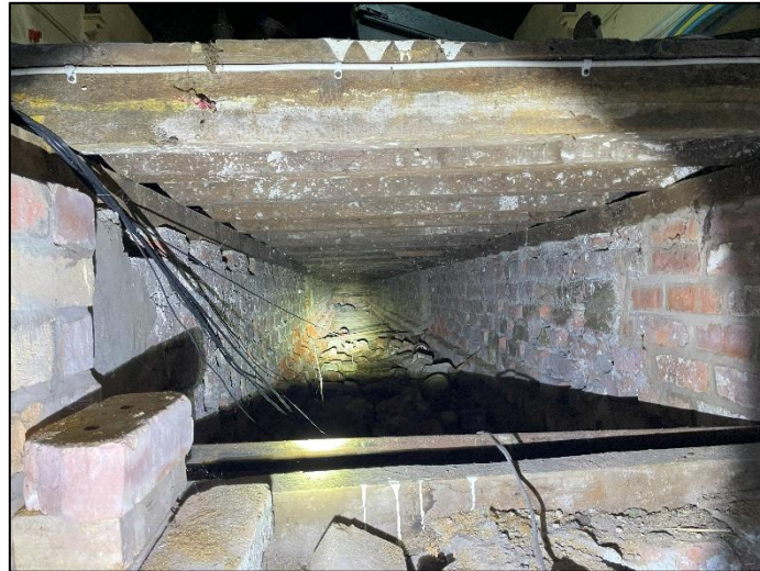
Figure 4.3 – Character of the foundations
