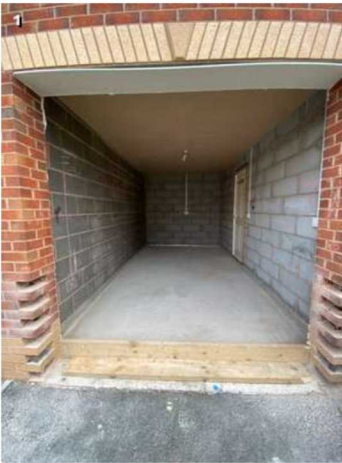
Garage with door removed
