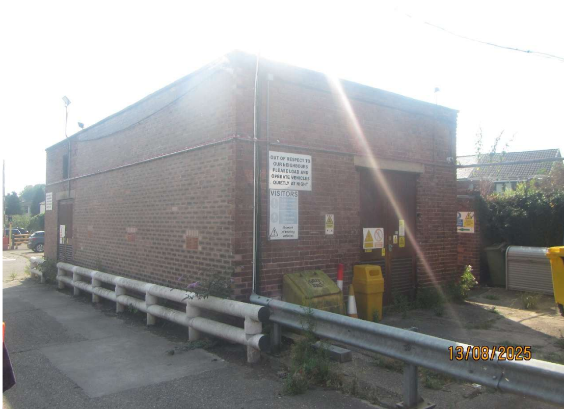
Photograph 6 – Example of a building onsite.
