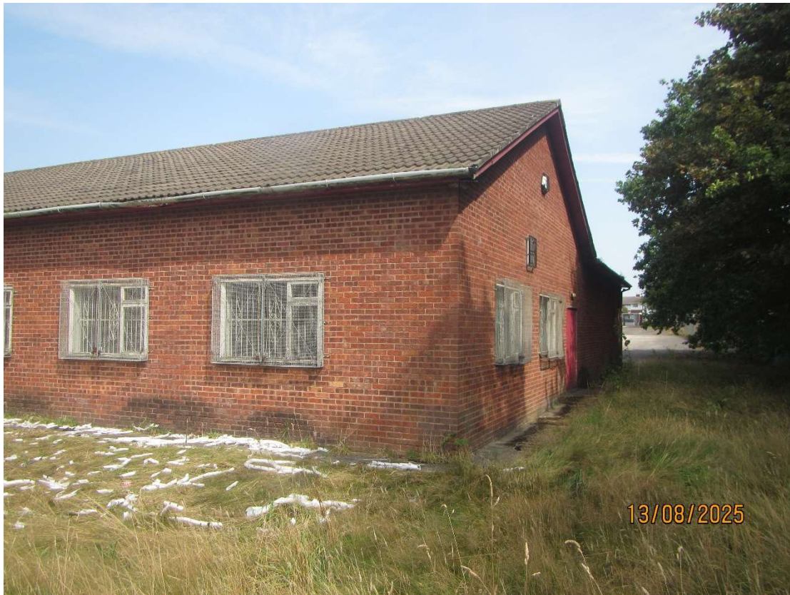
Photograph 5 – Example of a building onsite.
