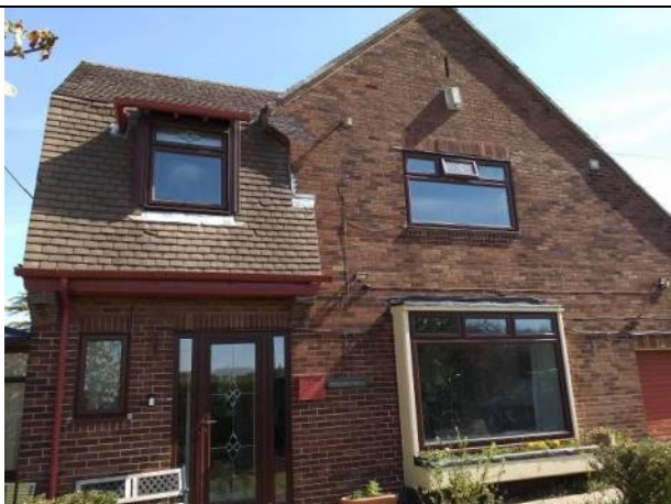
Photograph 7.6: Existing Dwelling (south-west elevation)
