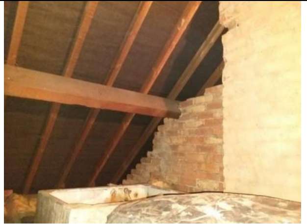
Photograph 7.8: Existing Dwelling Loft
