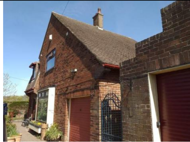
Photograph 7.7: Existing Dwelling (South-east elevation)
