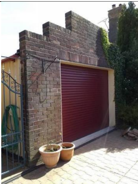
Photograph 7.10: Garage (South-east elevation)
