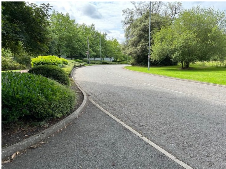
Photo 2.3: Existing 2.4m x 43m Visibility Splay (Trailing Traffic Direction)
