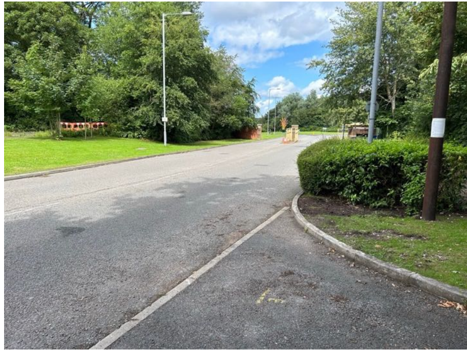
Photo 2.2: Existing 2.4m x 43m Visibility Splay (Leading Traffic Direction)
