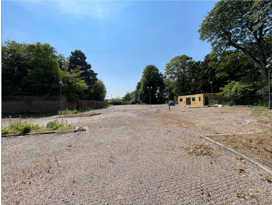
Image 1: Grade II Listed Garden Wall to the Hazels and temporary office structure
