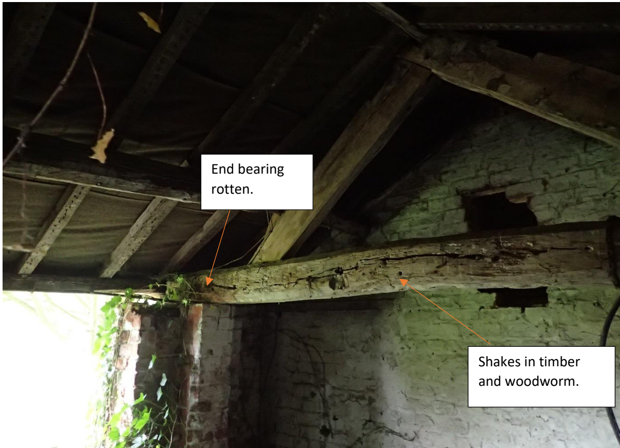
Photograph No. 5 – Detail of timber truss.
