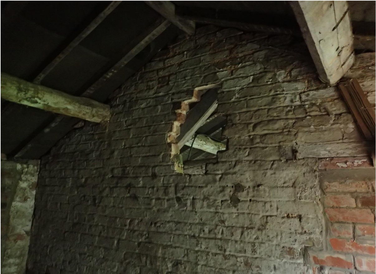
Photograph No. 7 – View of party wall with high level opening.
