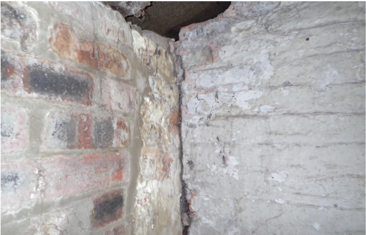
Photograph No. 2 – Unbonded corner detail side elevation and party wall.
