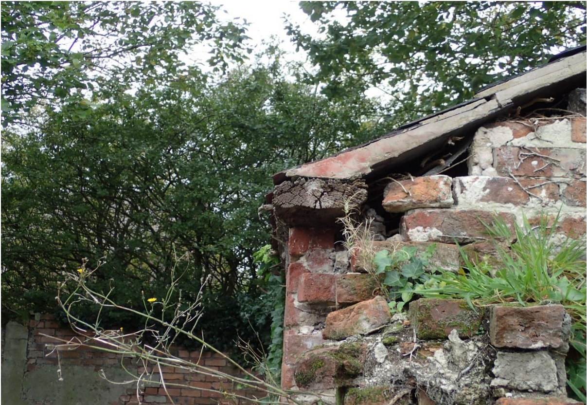
Photograph No. 9 – Detail at corner side/end gable at wall plate level.
