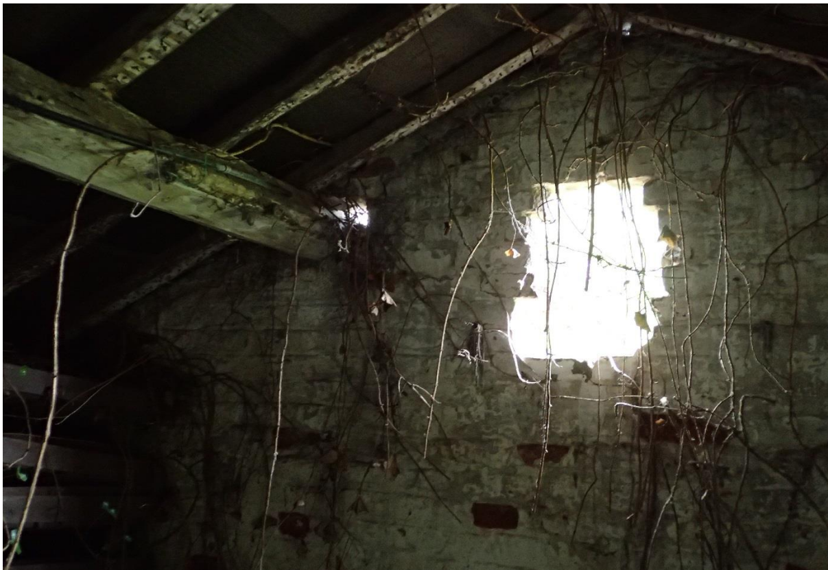
Photograph No. 6 – View of gable end with high level opening.
