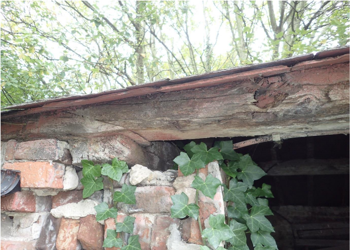
Photograph No. 3 – Detail of wall plate
