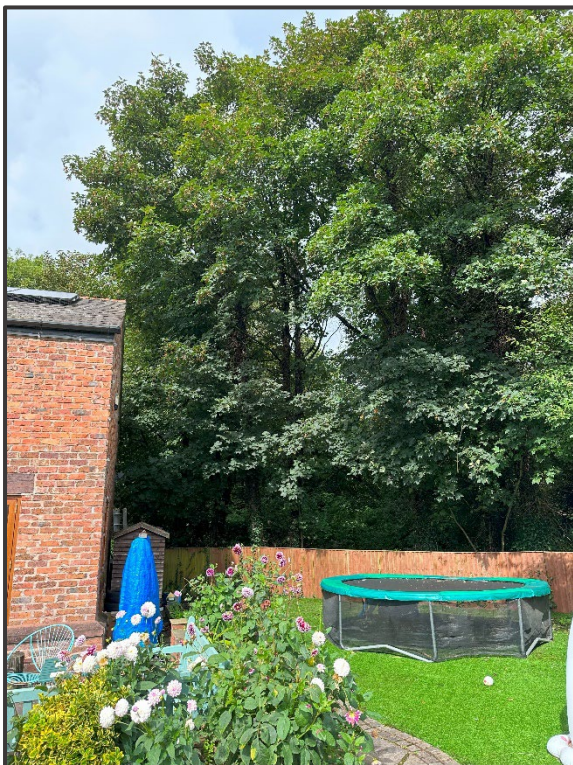
Picture 3. W1b to W1C. Note the Astro Turf area which will be compacted.
