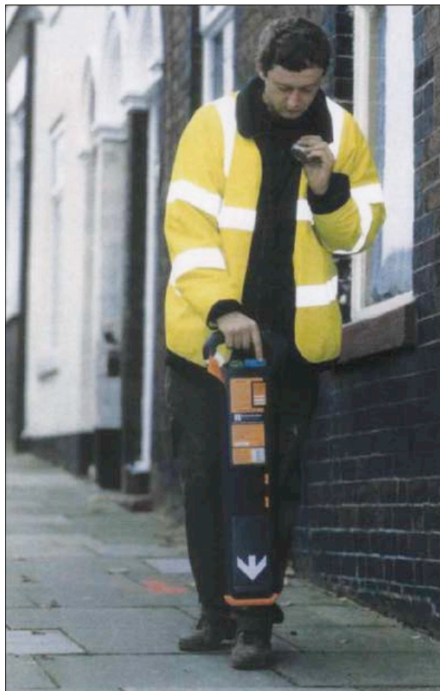
Figure 5 Using a cable locator
