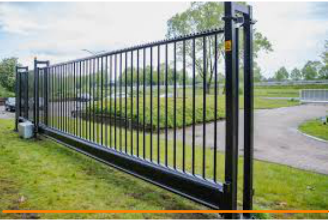
Example of Automatic sliding door into service yard
