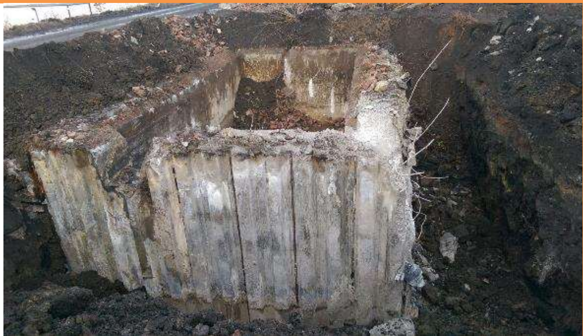
PLATE 7 – REMOVAL OF CONCRETE BELOW GROUND STORAGE TANK
