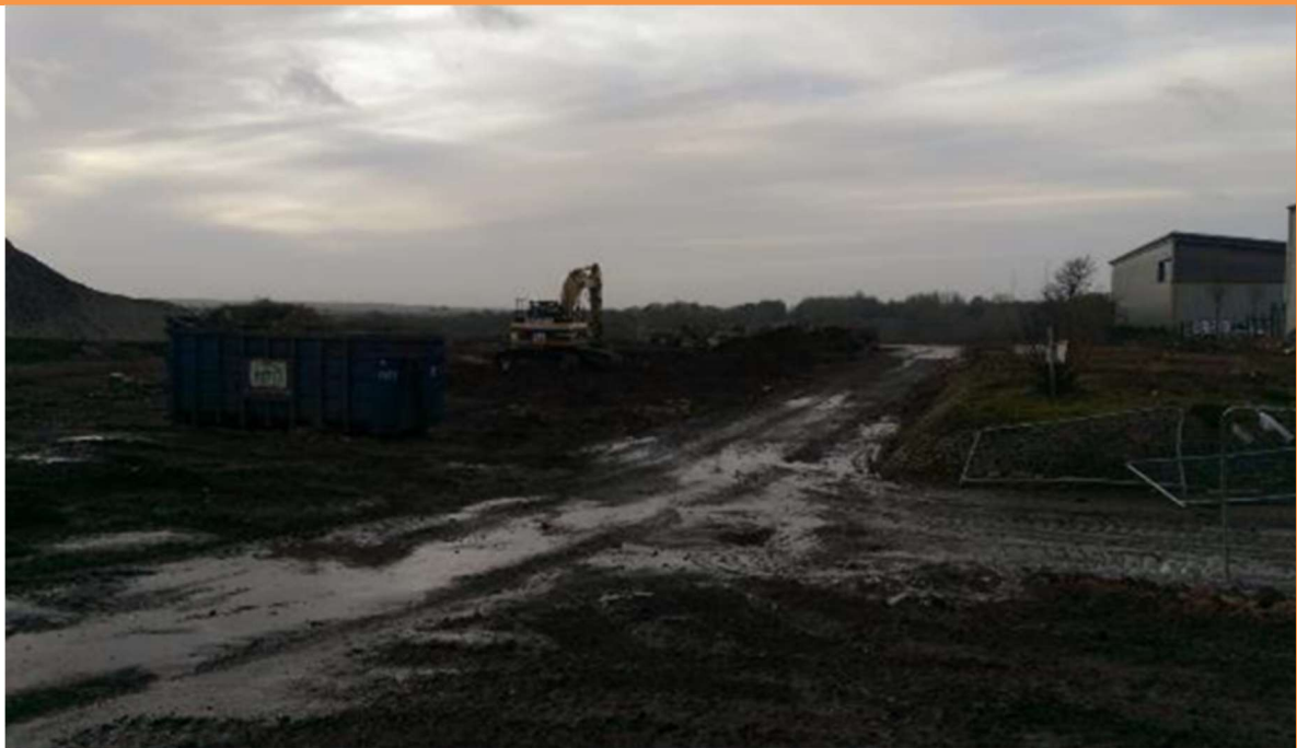
PLATE 5 – COMMENCEMENT OF REMEDIATION WITHIN UPPER AREA OF PARCEL C
