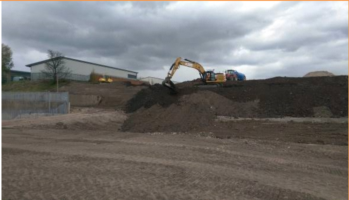
PLATE 20 – TURNOVER OF THE EMBANKMENT AFTER RETAINING STRUCTURES REMOVED
