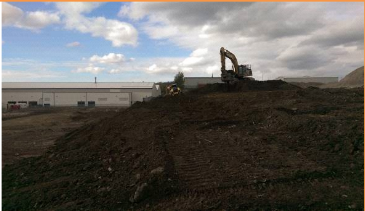
PLATE 23 – THE CENTRAL SECTOR OF PARCEL C BLENDING THE TWO SITE LEVELS INTO ONE
