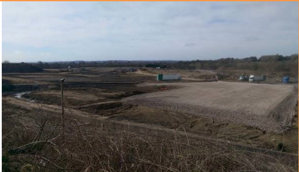
PLATE 17 – LOWER PARCEL C AFTER REMEDIATION SITE RAISING IN PROGRESS
