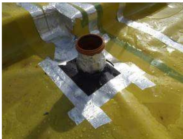
Photograph 4: Check top hat is sealed to membrane and pipework. If the formed top hat is not tight to the pipework then also confirm presence of jubilee clip beneath butyl tape.
