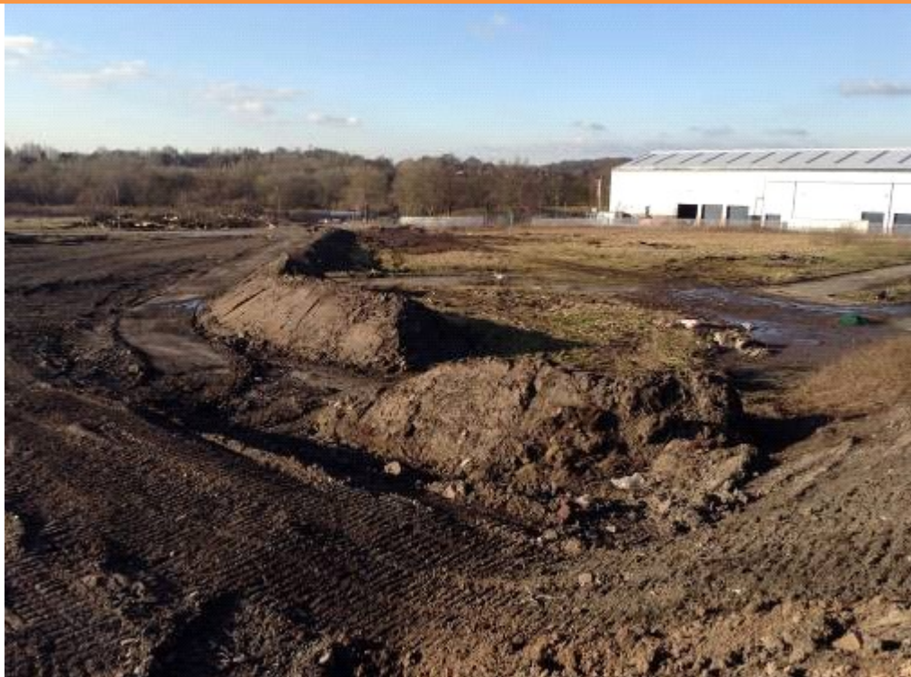
PLATE 2 – REMOVAL OF VEGETATION STRIP IN PROGRESS
