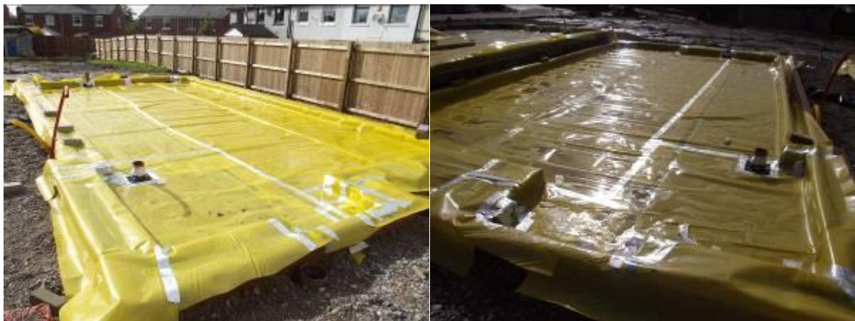
Photographs 1 and 2: Check general condition of membrane for punctures / tears etc
