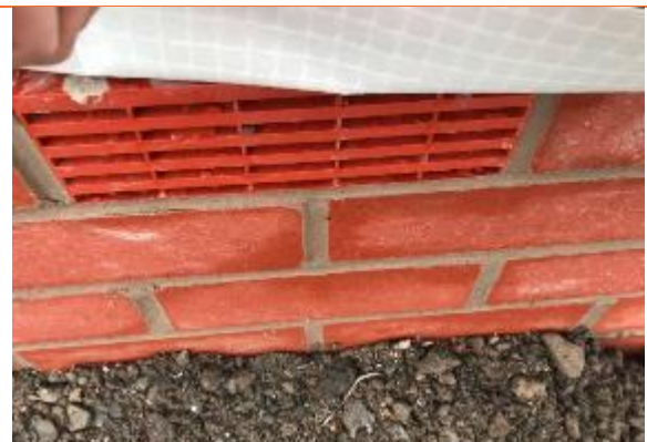
Verification of Service Penetrations-Good Condition
