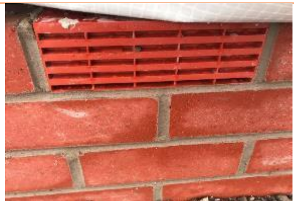
Verification of Service Penetrations-Good Condition
