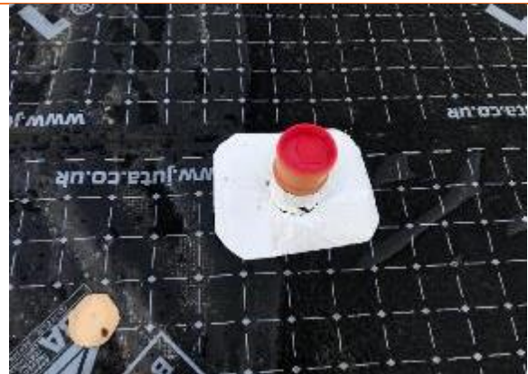
Verification of Service Penetrations-Good Condition
