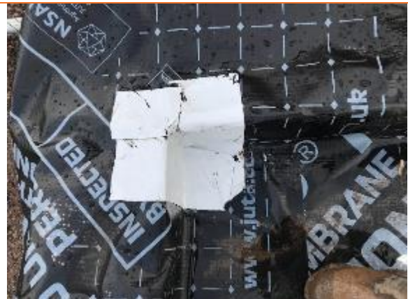
Verification of Service Penetrations-Good Condition
