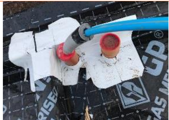
Verification of Service Penetrations-Good Condition
