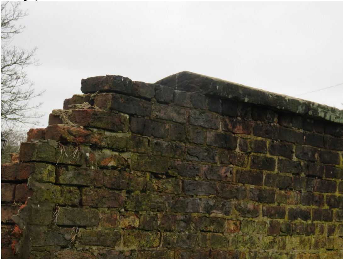
Handmade bricks to wall indicating the coursing and the red sandstone coping.
