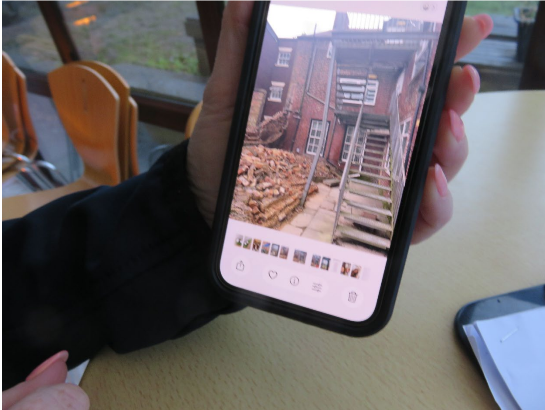
View taken from the adjoining owners of wall just shortly after collapsing.
