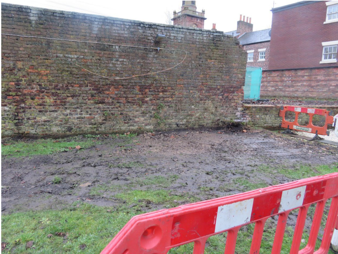
View of boundary wall from The Old Vicarage side indicating there is approximately 1.2 metres difference between the car park level and the vicarage yard level.
