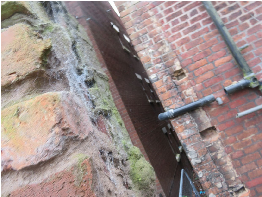
This shows the abutment of the wall where it ran into the rear wall of the original vicarage being bonded in every eighth courses.
