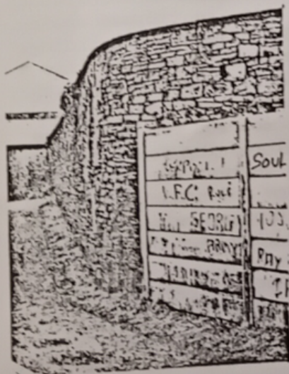
Wall 14 n-e corner.
