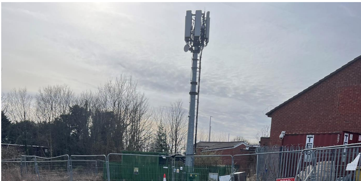
Figure 4 – Image of the telecommunications mast on site
