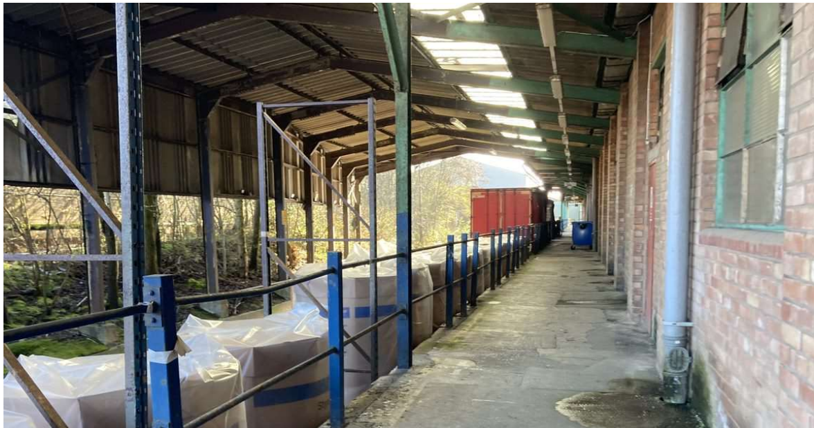
PLATE 4 SHELTERED SERVICE ROAD ALONG NORTHERN BOUNDARY (FACING NORTHEAST)
