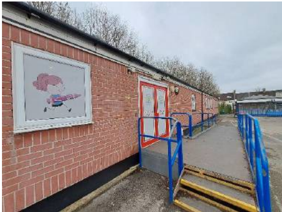
Photograph 3: Western aspect of building B1 (photograph taken facing south)
