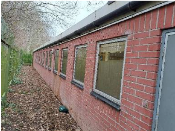
Photograph 7: Eastern aspect of building B1 (photograph taken facing south)
