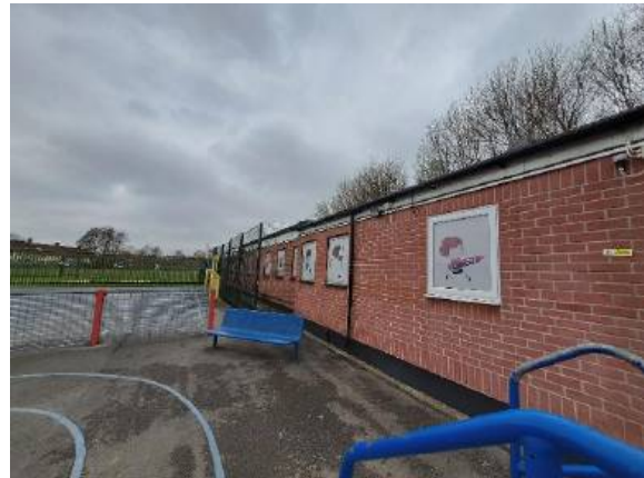
Photograph 4: Further example of western aspect of building B1 (photograph taken facing north)
