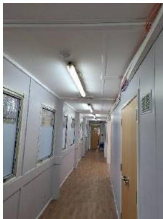
Photograph 9: Example of internal building condition (corridors)
