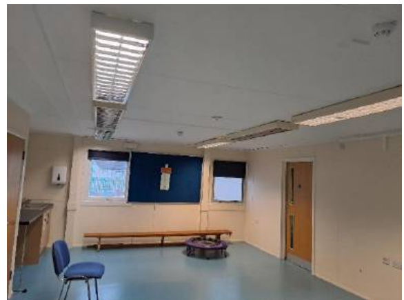
Photograph 10: Example of internal building condition (classrooms)
