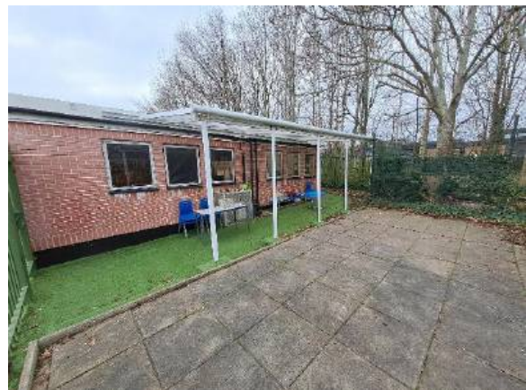
Photograph 6: Southern aspect of building B1 and further example of hardstanding (paving) present within the site
