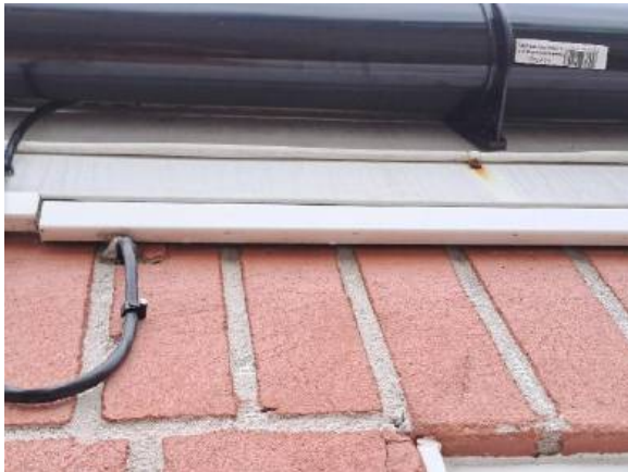
Photograph 11: Example of well-sealed fascias present throughout building B1
