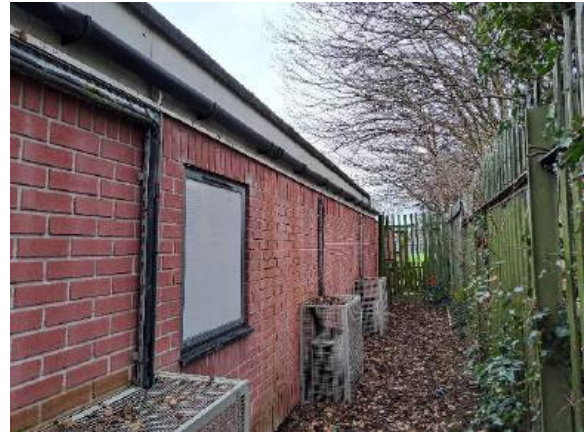
Photograph 8: Further example of eastern aspect of building B1 (photograph taken facing north)
