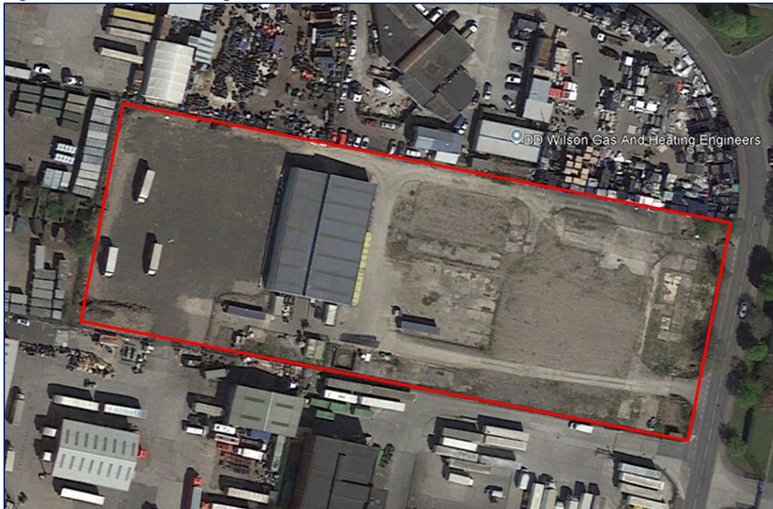
Figure 2: Site Aerial Image
