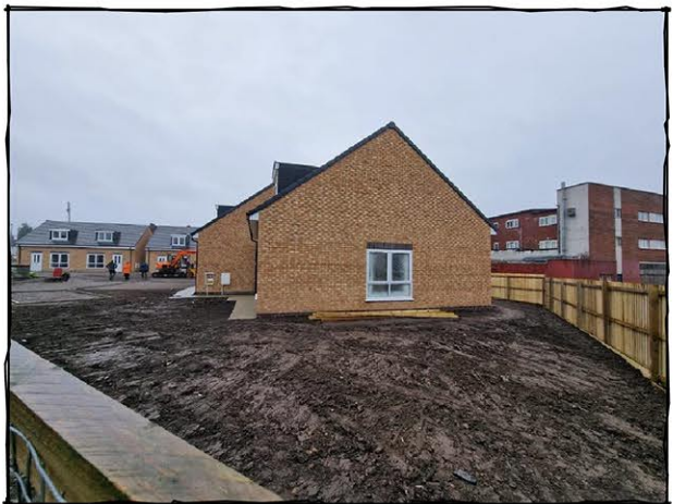
Photo 2 - End Gable of Unit 9
