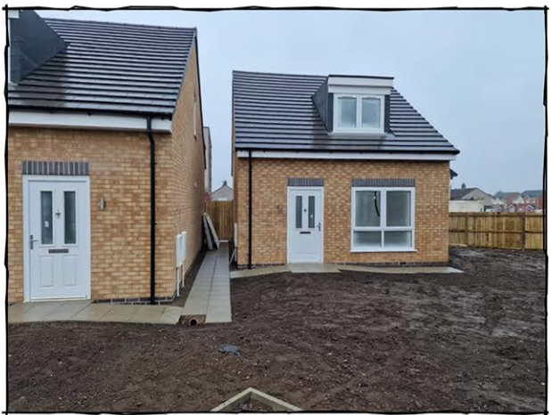
Photo 3 - Front View of Unit 8 & 9
