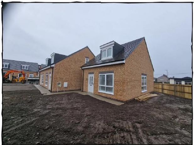
Photo 4 - Corner View of Unit 9
