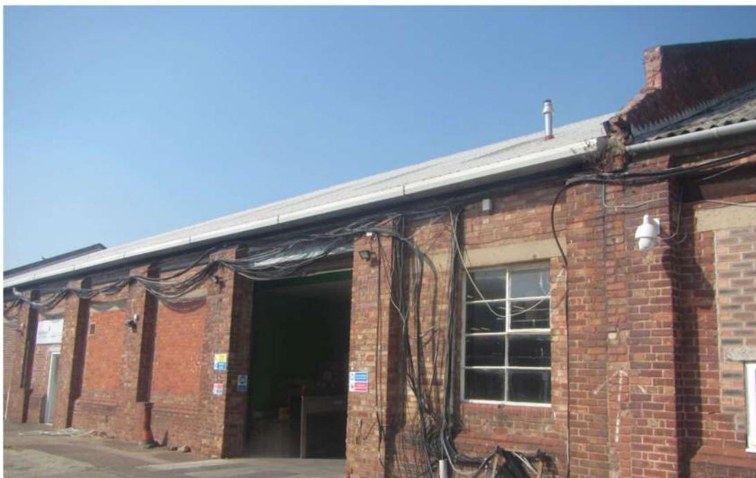
Photograph 4 – Sheet metal roof on Building 1.
