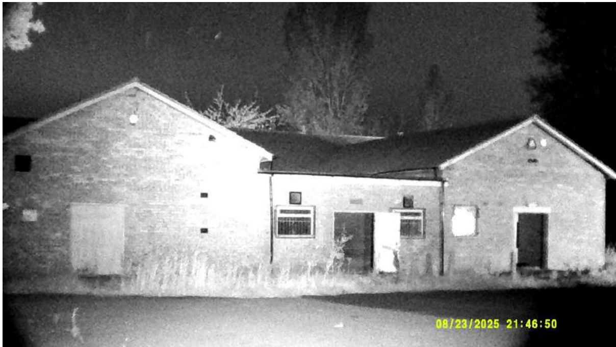
Photograph 5 – Infrared image taken of the aspect of Building at the darkest point of the survey at on.
