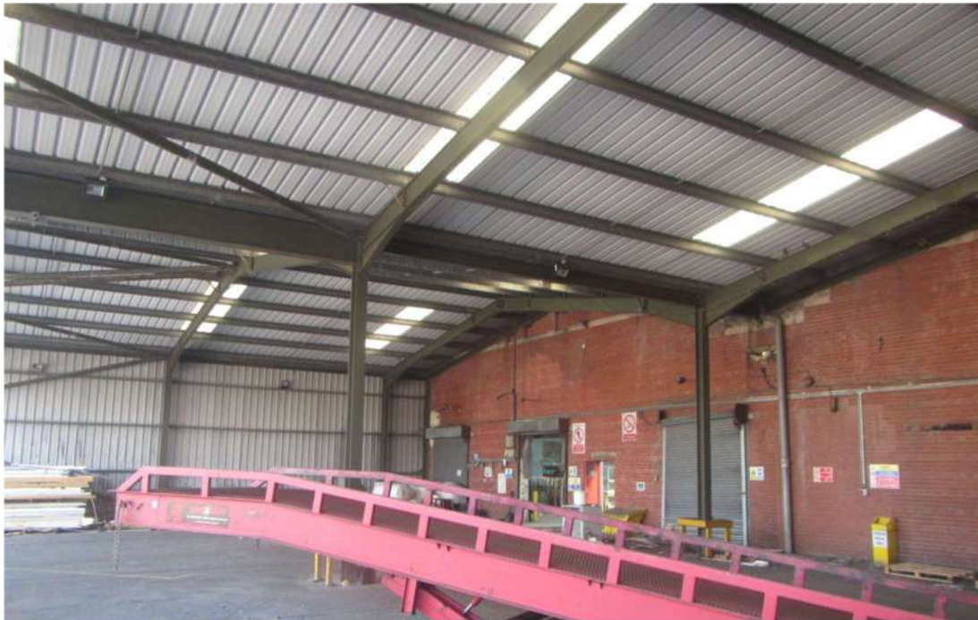
Photograph 19 – Large open interior of Building 1.
