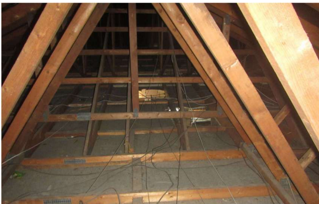
Photograph 22 – Traditional timber rafter and purlin structure within Building 7.
