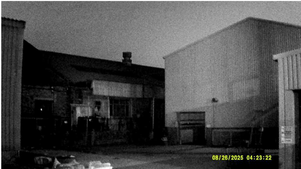
Photograph 9 – Infrared image taken of the northern aspect of Building 1 at the darkest point of the survey at 04:23 on 26 th August 2025.
