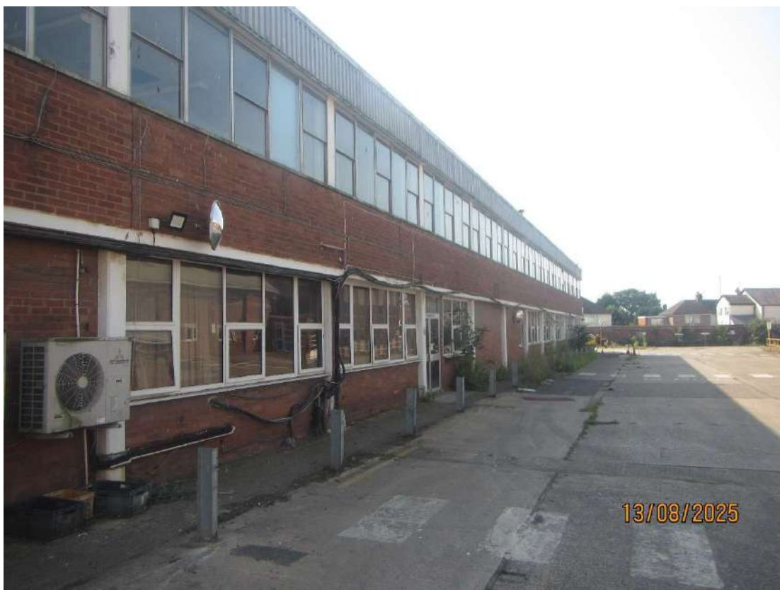
Photograph 10 – The northern aspect of Building 2.
