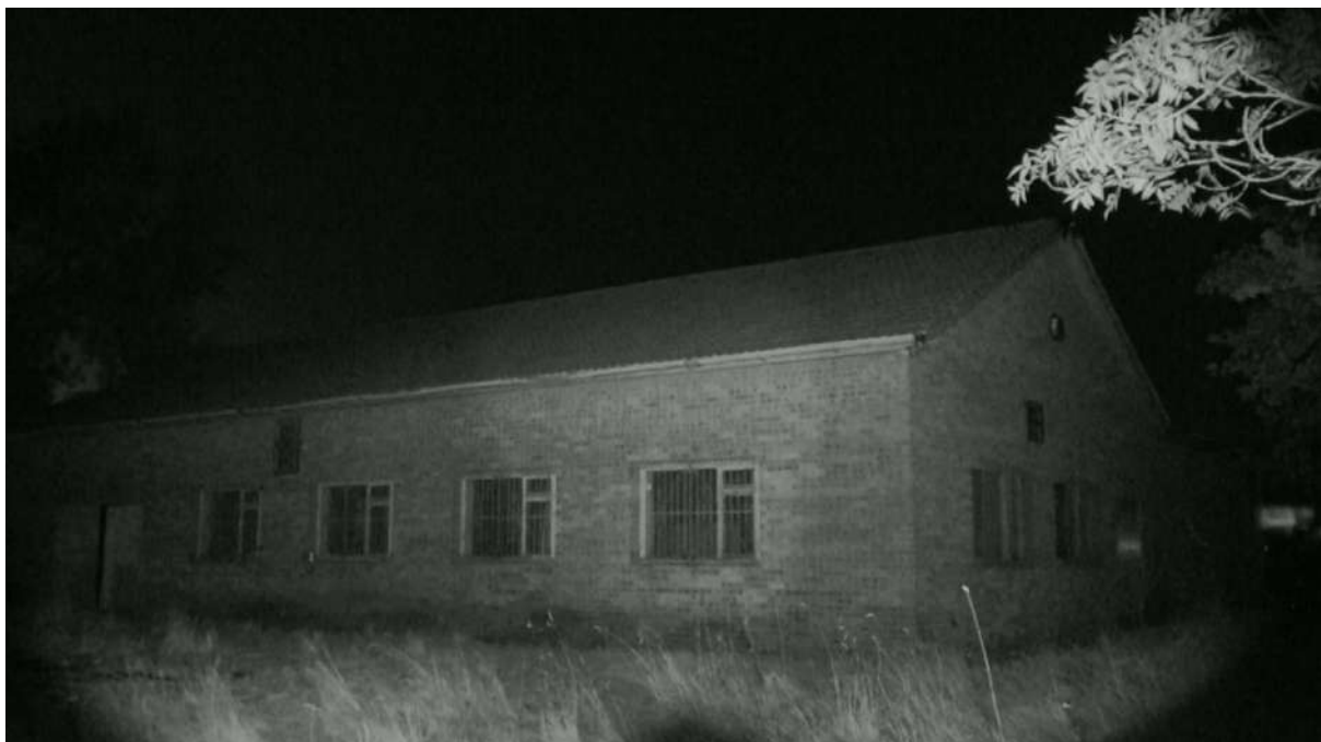
Photograph 14 – Infrared image taken of the southern aspect of Building 7 at the darkest point of the survey at 20:32 on 25 th September 2025.
