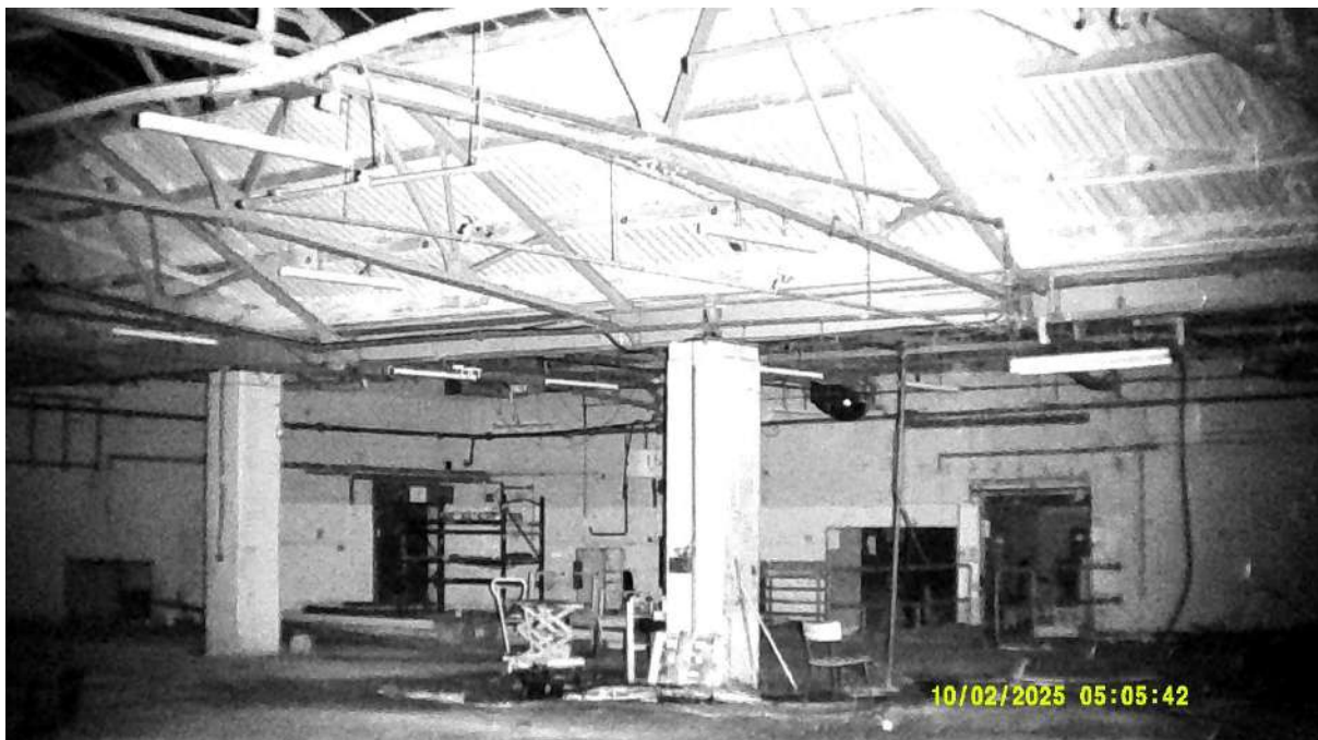
Photograph 22 – Infrared image taken of the aspect of the western interior of Building 1 at the darkest point of the survey at 05:05 on 2 nd October 2025.
