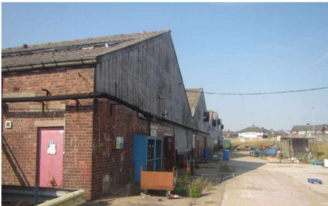
Photograph 1 – The eastern aspect of Building 1, showing the pitched roofs.
