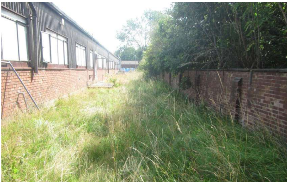
Photograph 12 – The southern aspect of Building 3 which is constructed of red brick with asbestos cladding.
