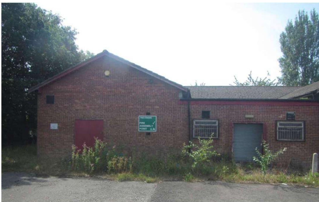
Photograph 15 – Building 7 which contains a multi-pitched roof and external redbrick walls.
