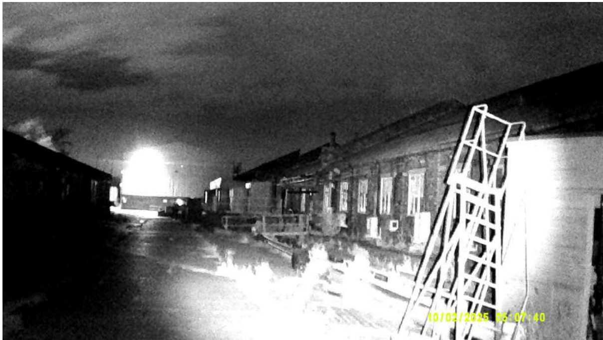
Photograph 23 – Infrared image taken of the southeastern aspect of Building 1 at the darkest point of the survey at 05:07 on 2 nd October 2025.
