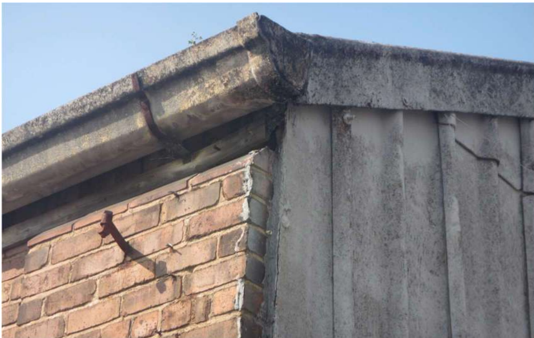
Photograph 6 – Wooden fascia boards located along the eaves of Building 1.
