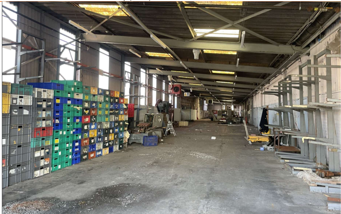
PLATE 04 Former Aluminium Shop (North)
