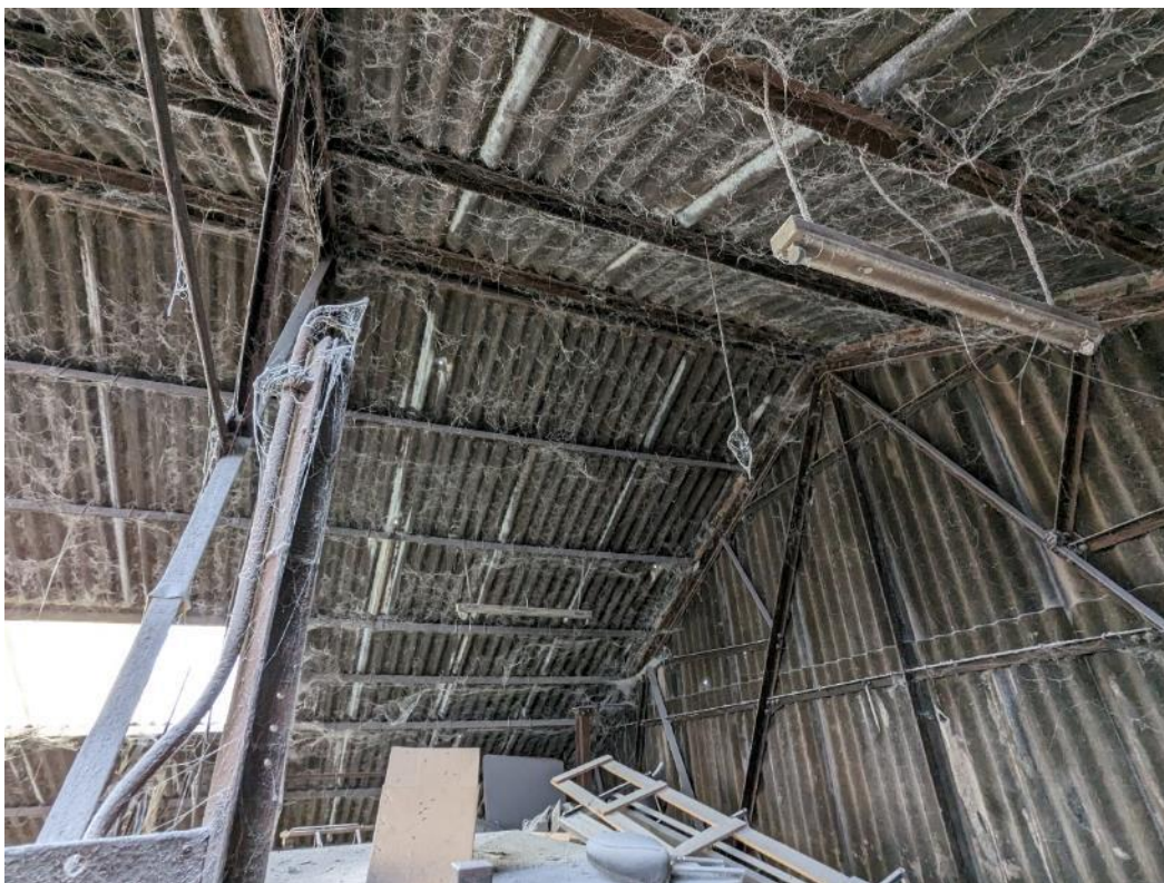
Plate 2 – Nature of the underside of the roof cover inside B1
