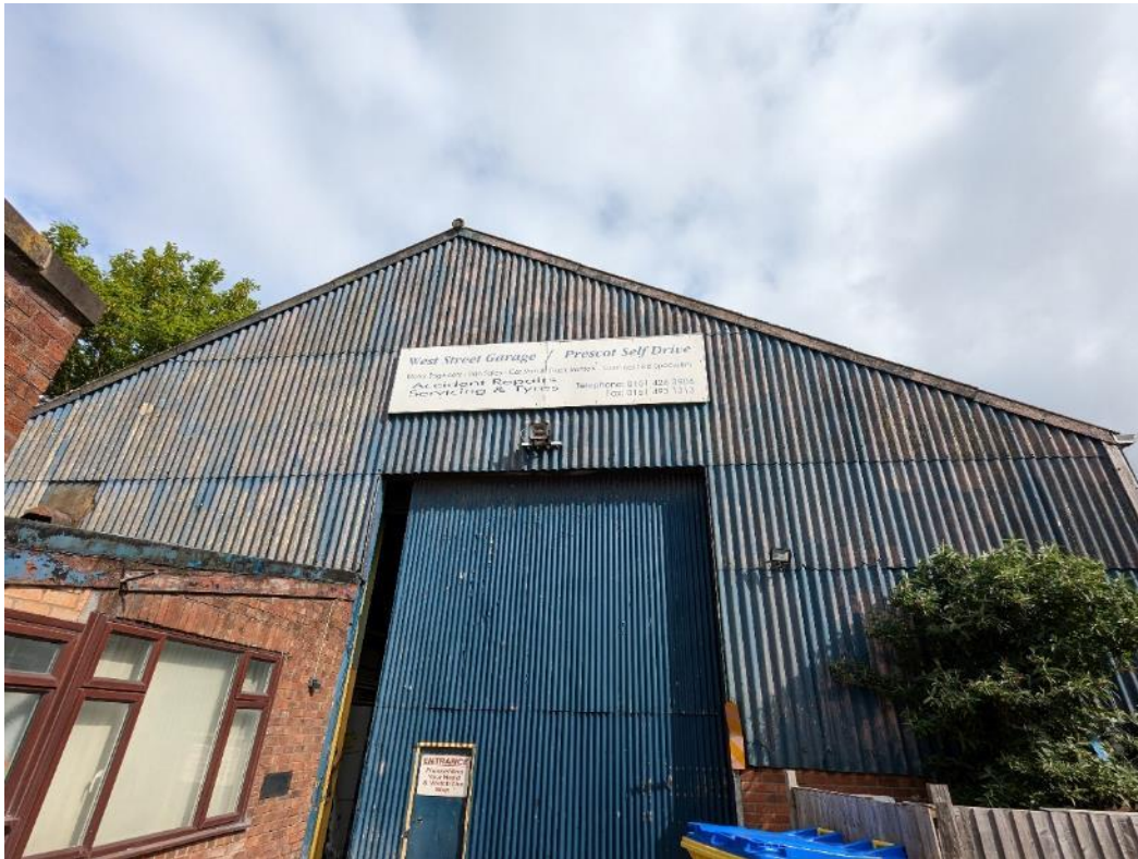
Plate 1 – Front south elevation and entrance of B1
