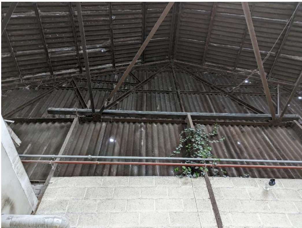
Plate 4 – Interior of B1 inner rear gable
