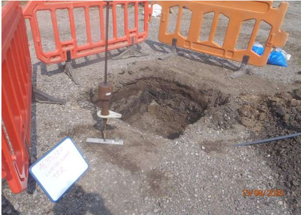
PHOTO 3 SHOWING GENERAL SOIL PROFILE AND POSITION OF DCP
