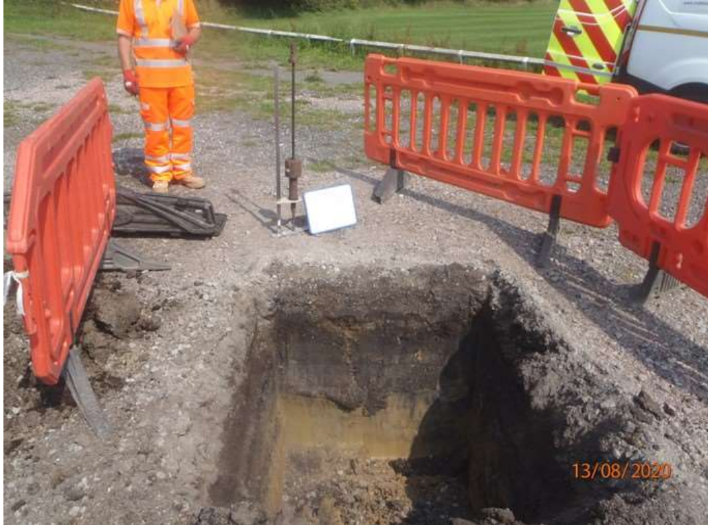
PHOTO 6 SHOWING SOAKAWAY LEVEL ON 2nd DAY
