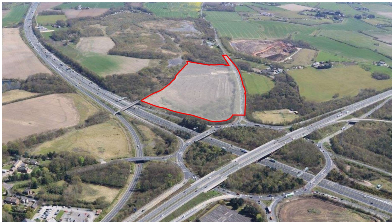
Fig.1b- Aerial View Looking South East toward the site
