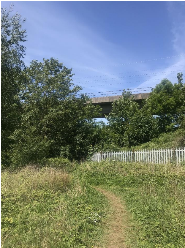
Figure 15. View west, at start of Phase 5.
