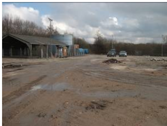
Northeast corner showing fire tank, asbestos roof and formerly vertical tanks, waiting for disposal
