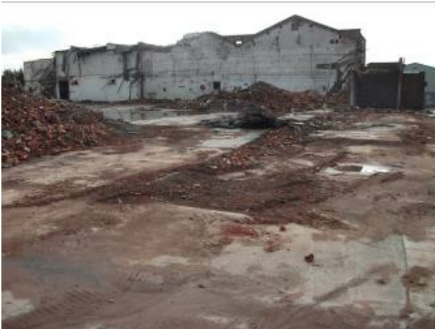
Demolished main building with floor intact
