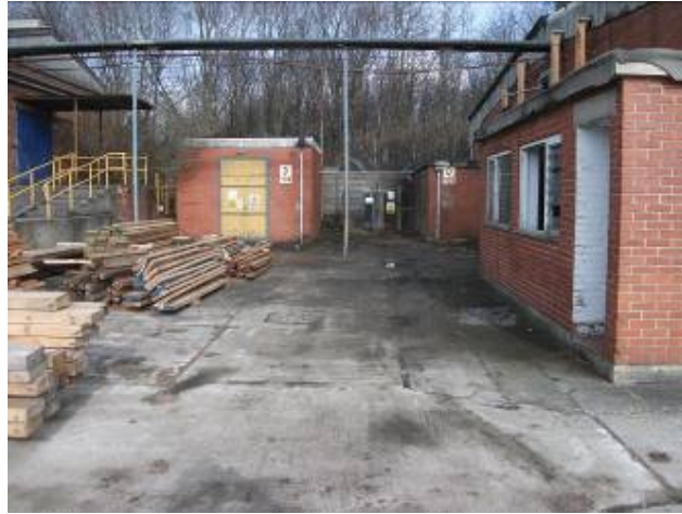
Transformer with Sub-station on left
