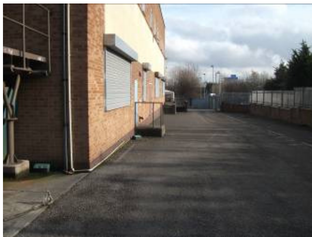
Offices fronting onto Allis Ashton Street
