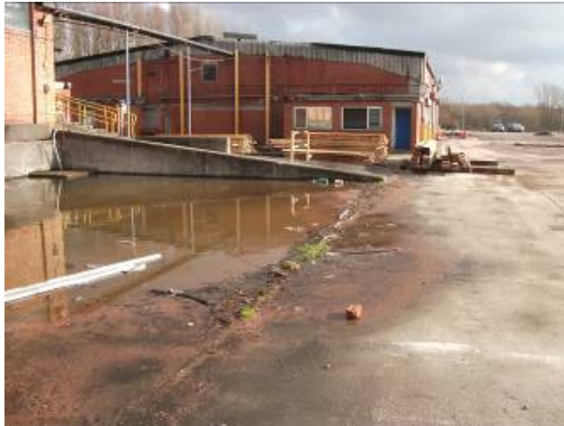
Washdown area with sump in left corner
