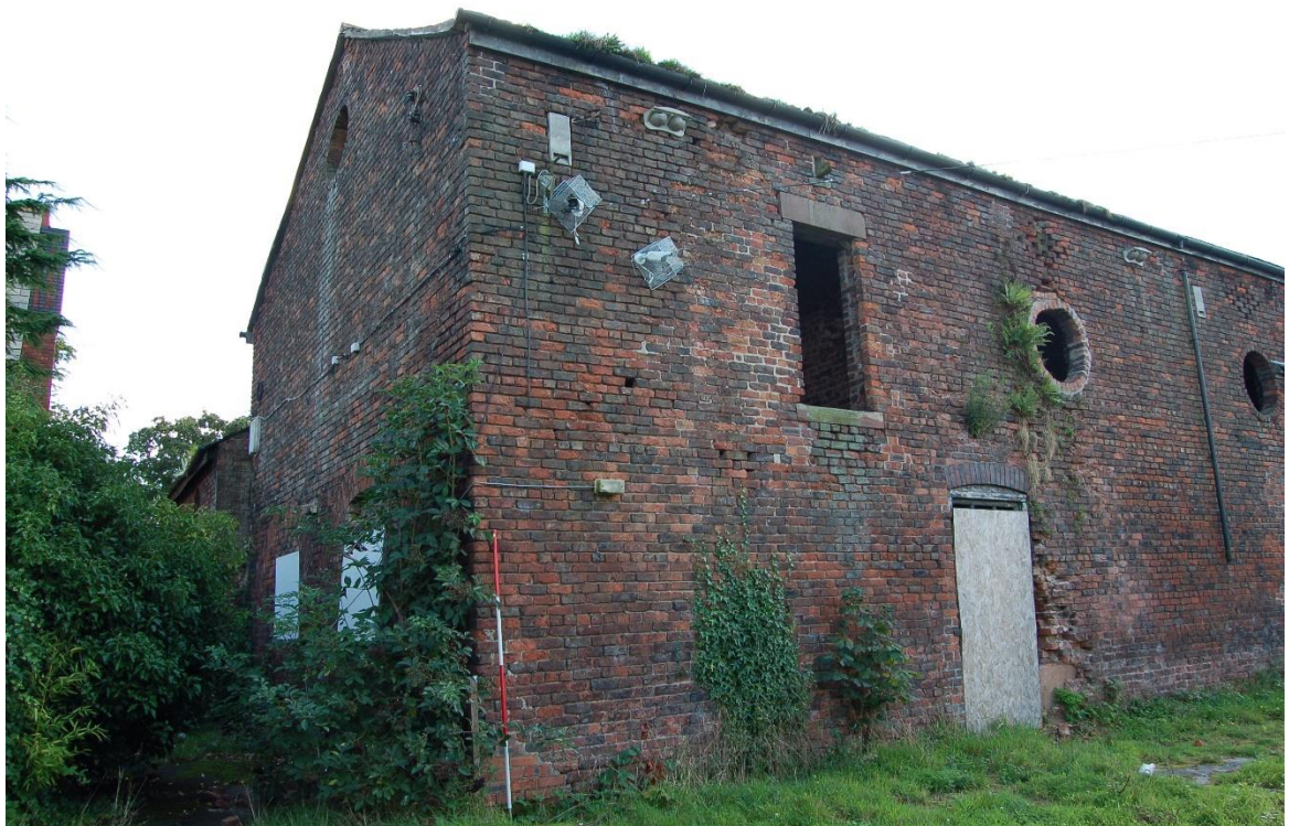
4. East facing elevation, and north facing elevation (eastern end)
