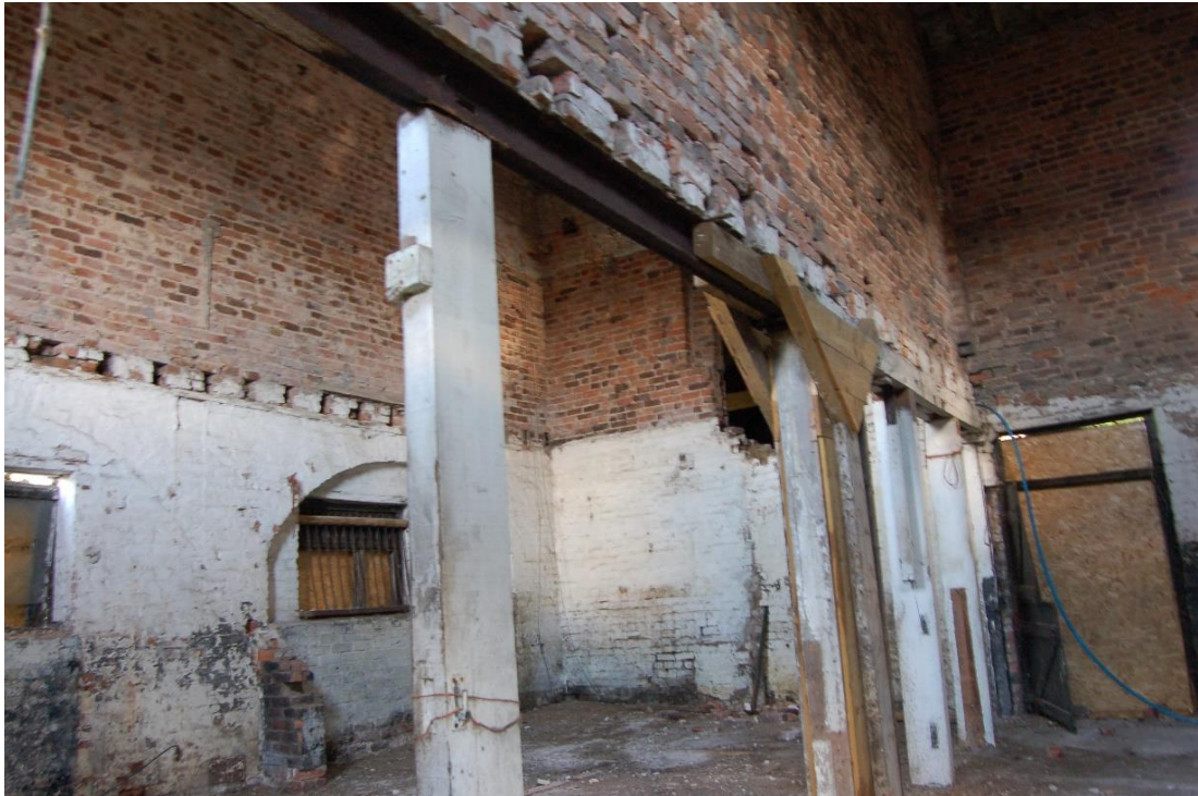
Interior main barn (showing bays and arches in east facing elevation)
