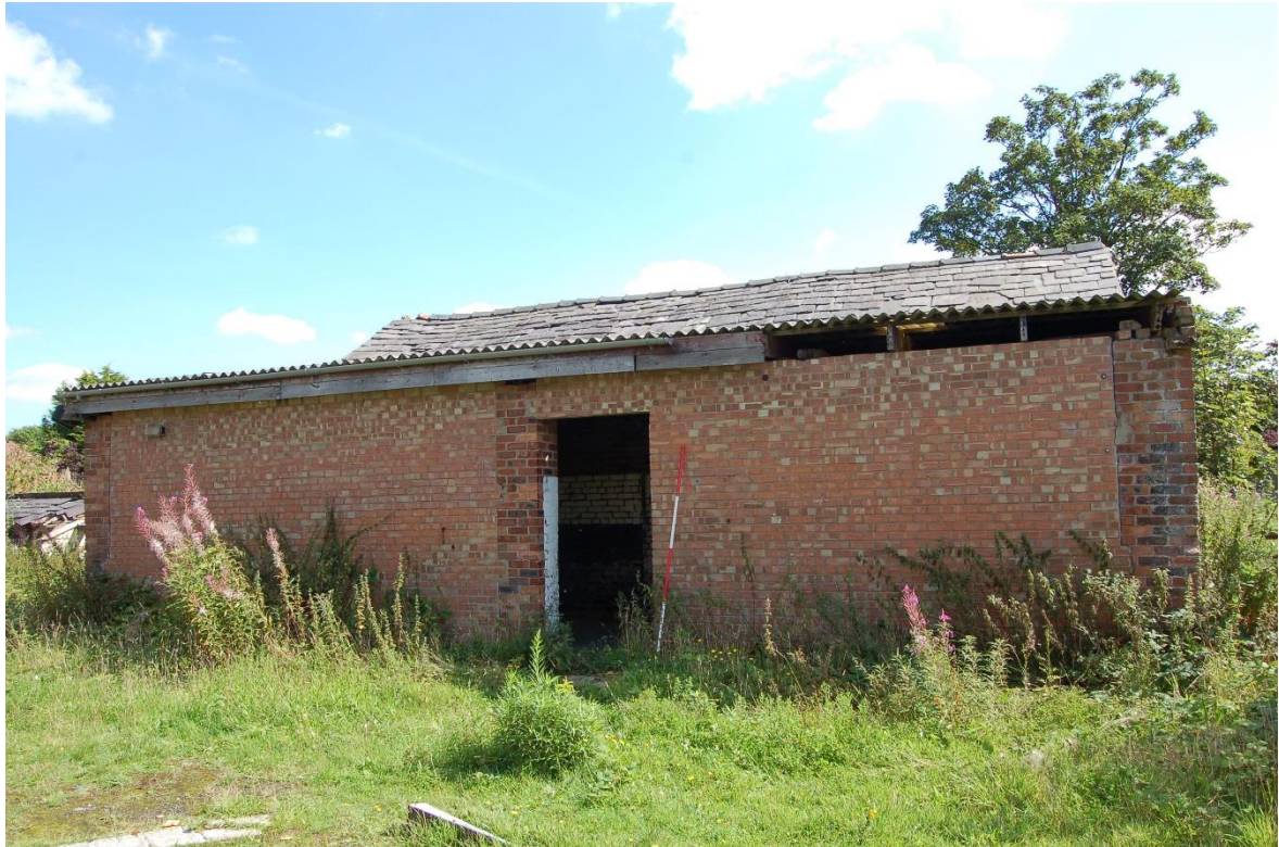
17. North facing elevation of storage barn (modern lean-to extension)
