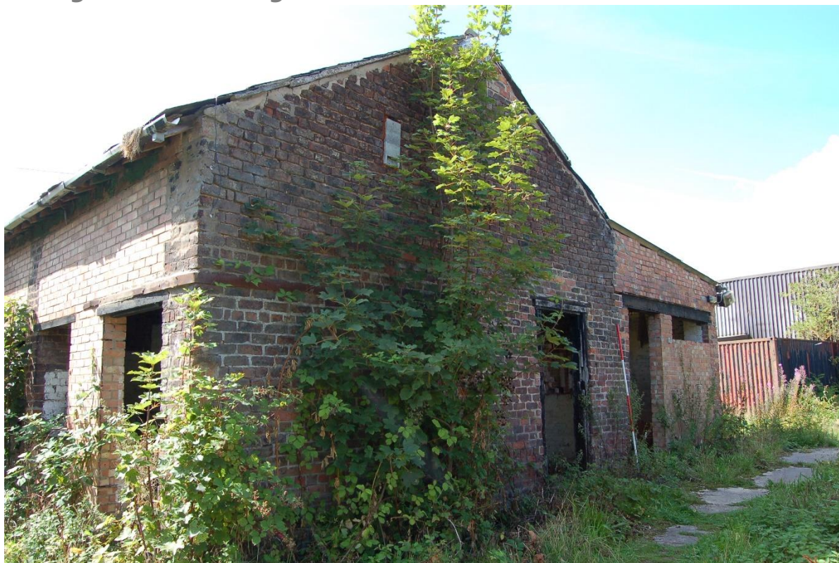
15. East facing elevation of storage barn
