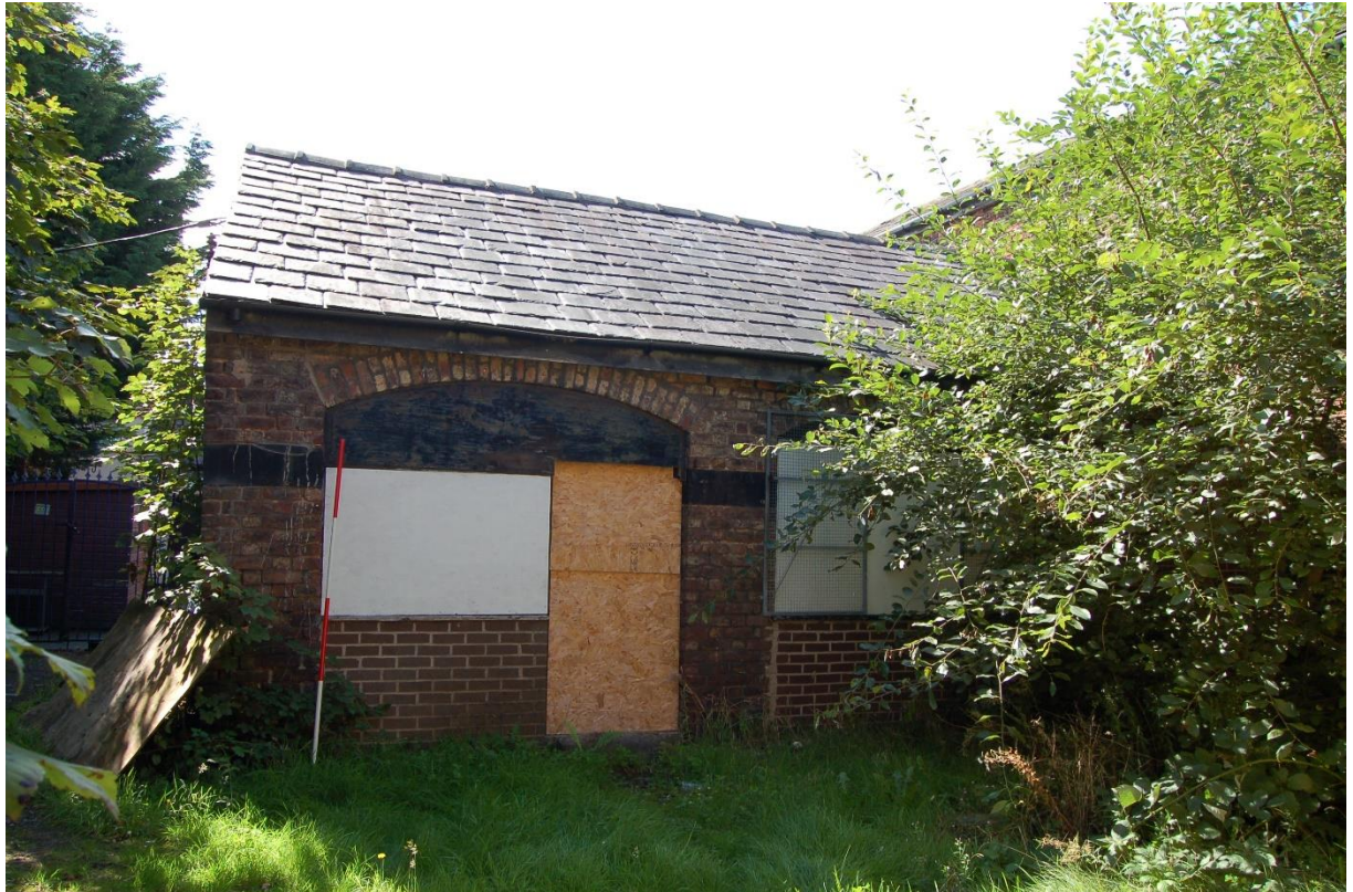
3. Main barn, east facing elevation of middle adjoining single storey barn (F8B)
