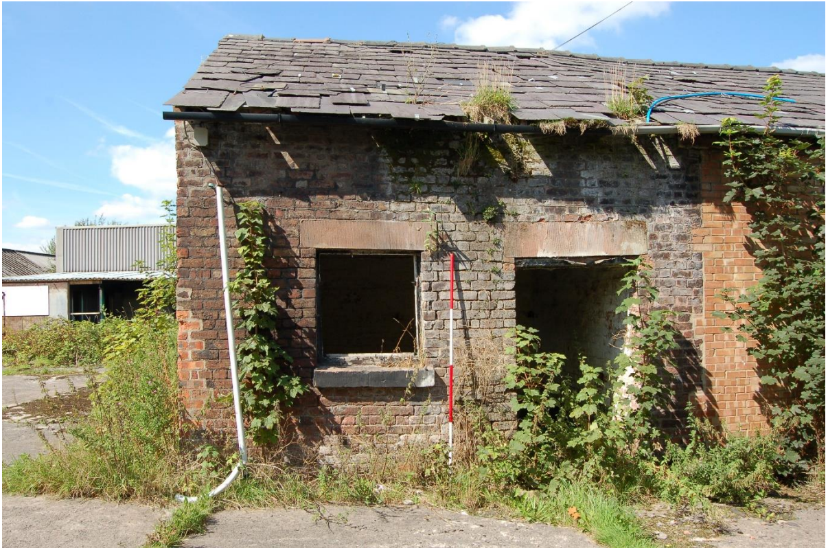
19. South facing elevation of storage barn
