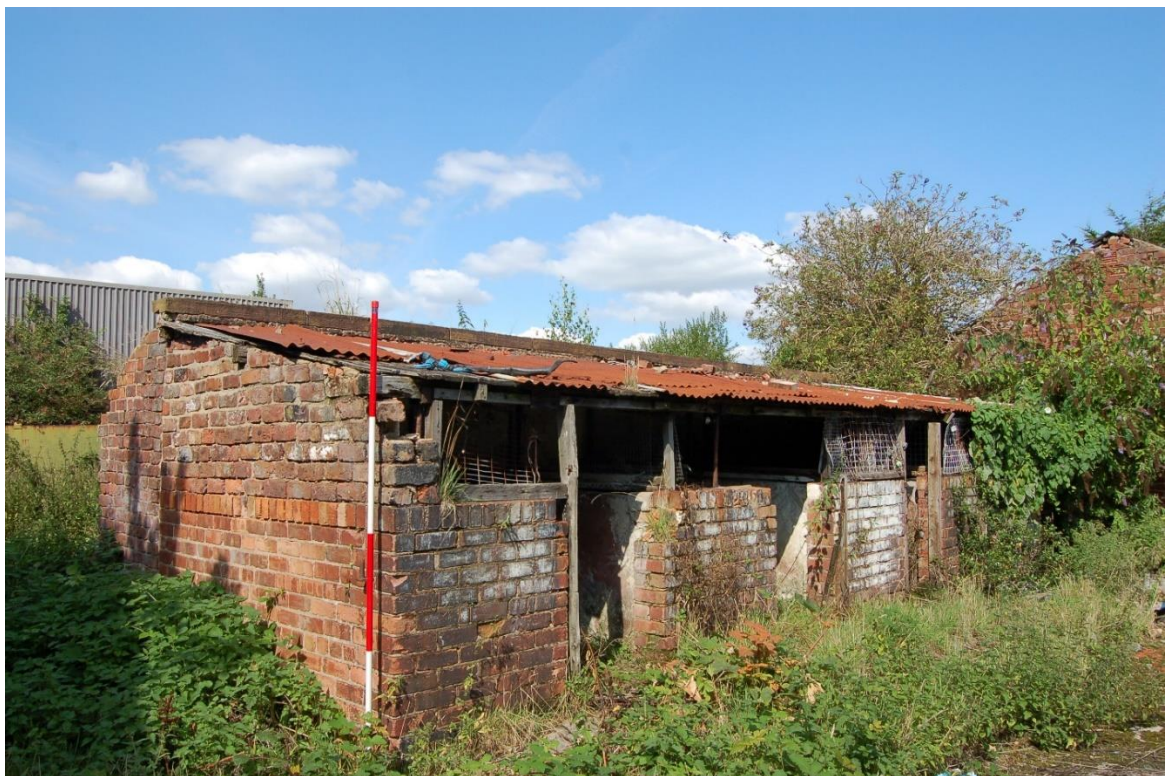
12. South and west facing elevations of pigsty
