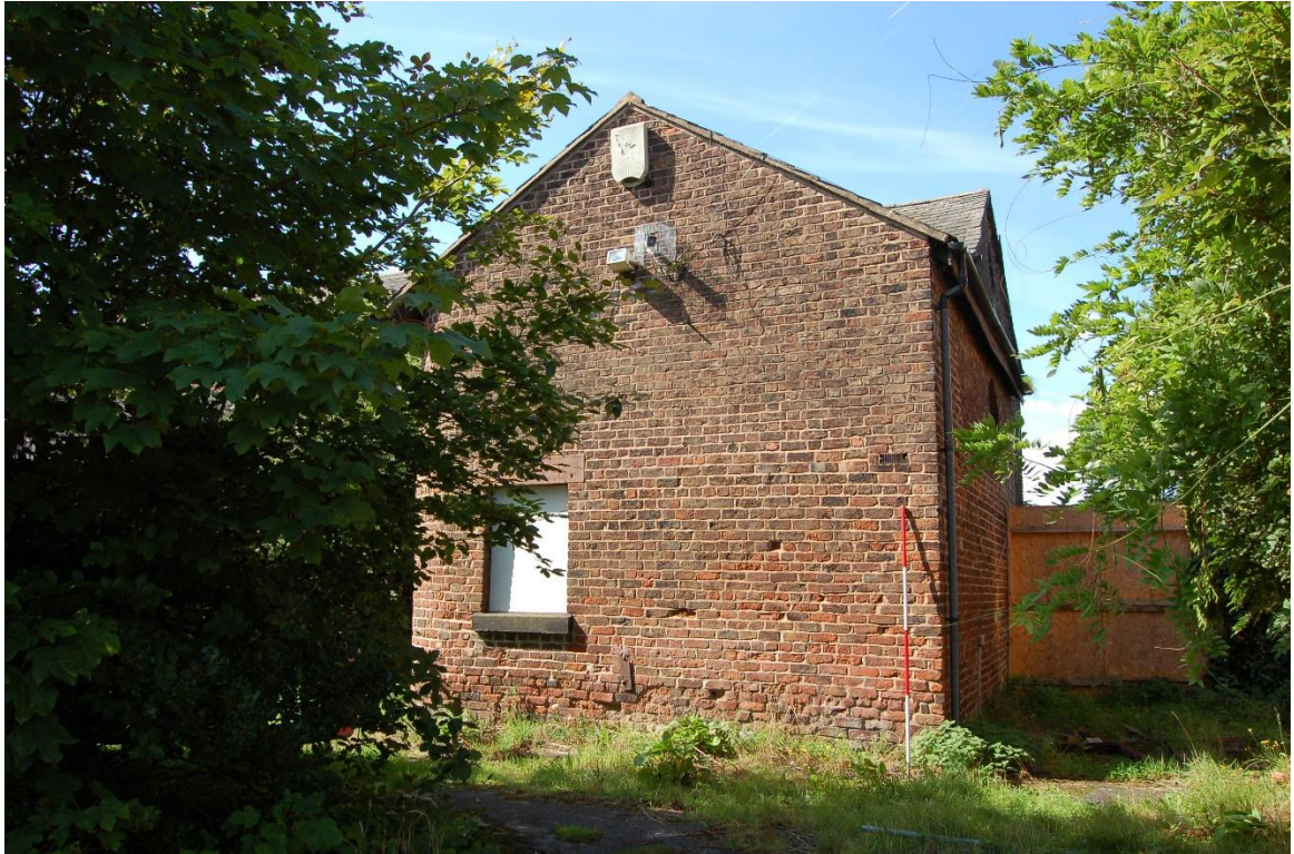
1. Main barn, south facing elevation of south-eastern adjoining single storey barn (F8D)
