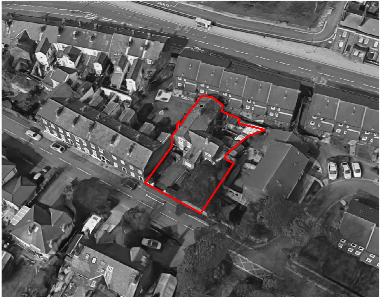
Aerial image of No.10 West Street
