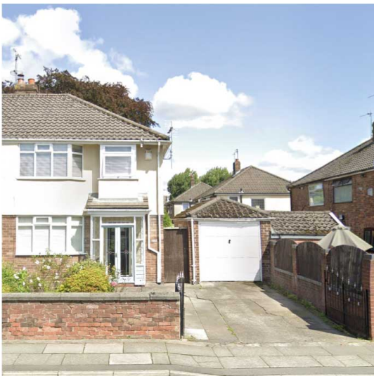
IMG_02 (L): Front elevation 215 Tarbock Road (source: google)
