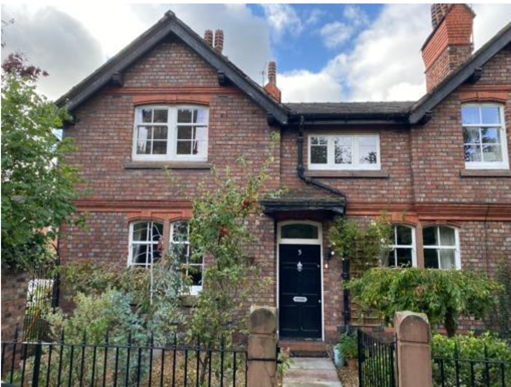
Photo 2 - Face brick, band courses, sandstone cills, sliding sash windows, slate roof
