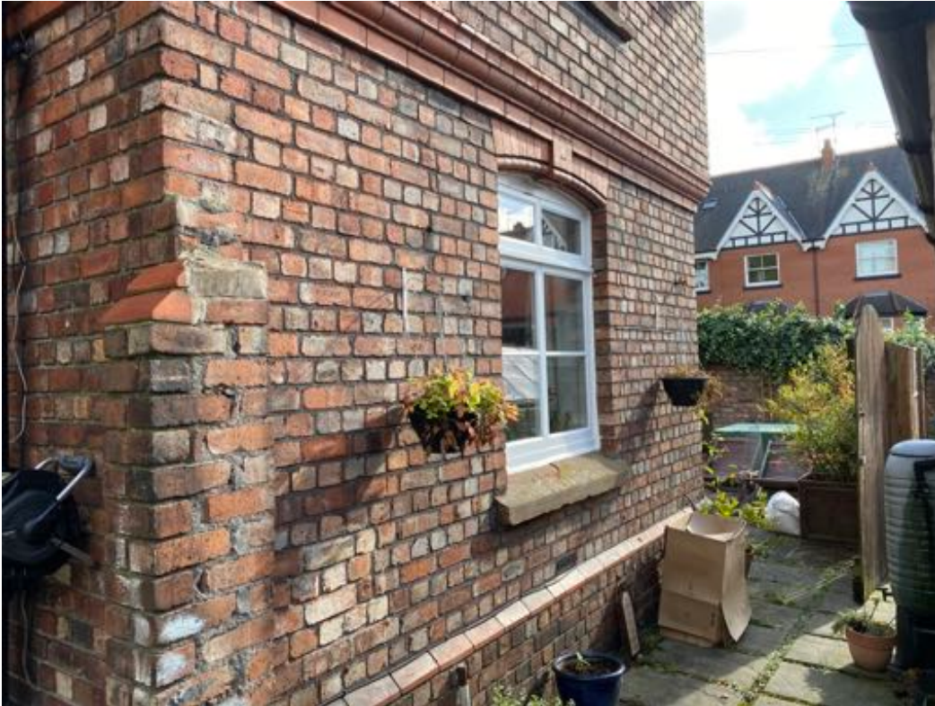
Photo 2 - Face brick, band courses, sandstone cills, sliding sash windows, slate roof
