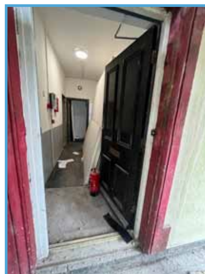
Existing side entrance door
