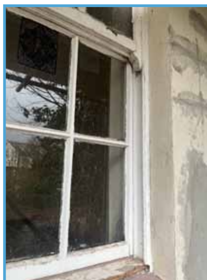
Existing sash windows
