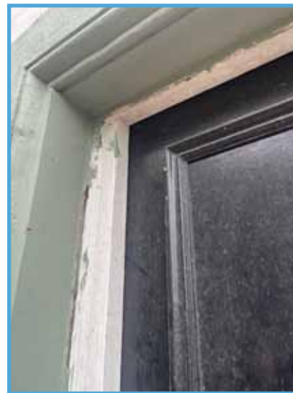
Existing 1980s side entrance door. Ply faced fire door with planted on softwood beading to form panels The cill is placed directly upon the facing brickwork
