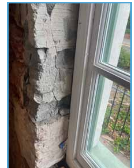
Example of 1980s workmanship to infill window sash with lightweight blockwork
