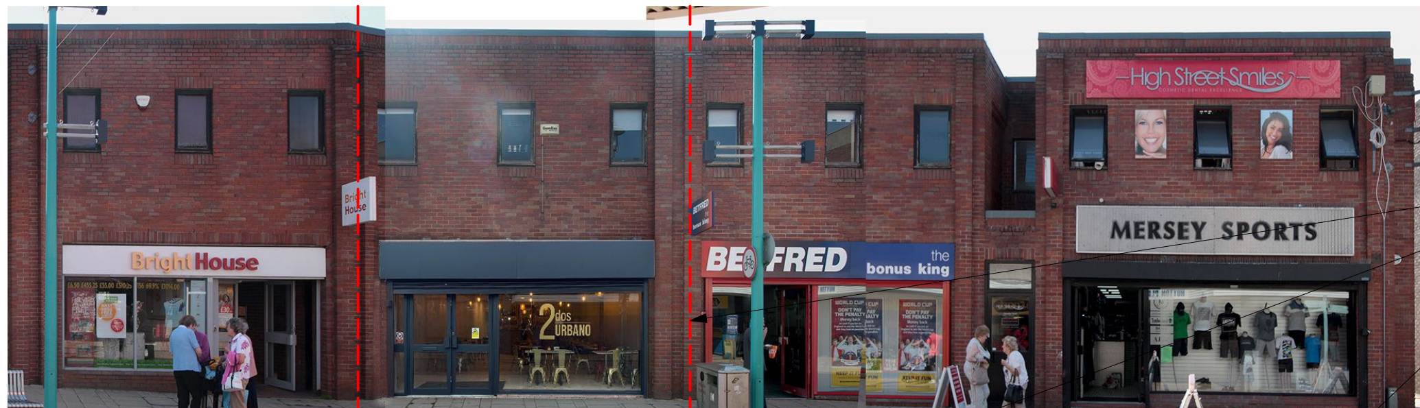
EXISTING PHOTO SURVEY
