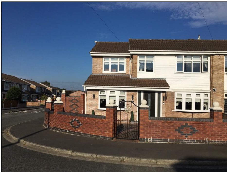
Figure 4: No.1 Mulberry Close, showing limited visual amenity impact of two storey side extension on corner plot
