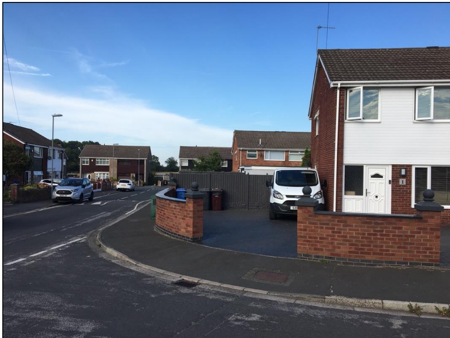
Figure 2: No.1 Dee Close with inset from rear property, due to differential building lines
