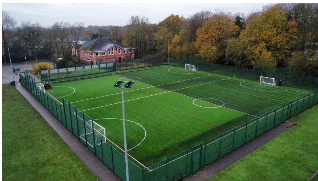
An example of a small sided AGP with 10m high floodlighting columns.
