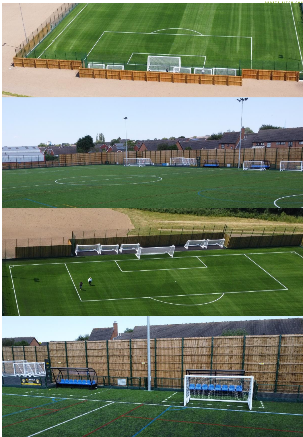
Examples of perimeter acoustic fencing
