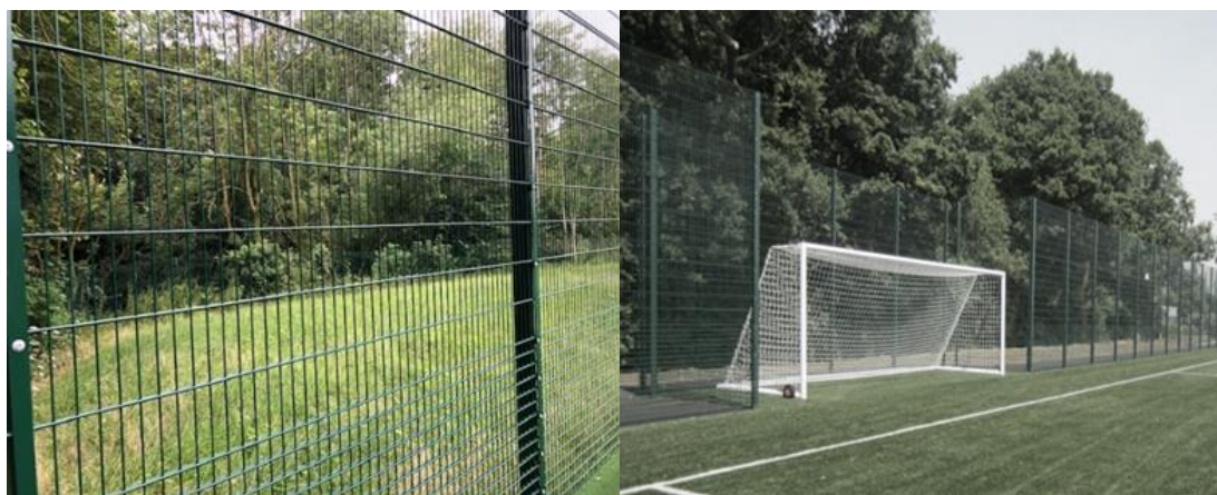
Examples of perimeter ball stop fencing
