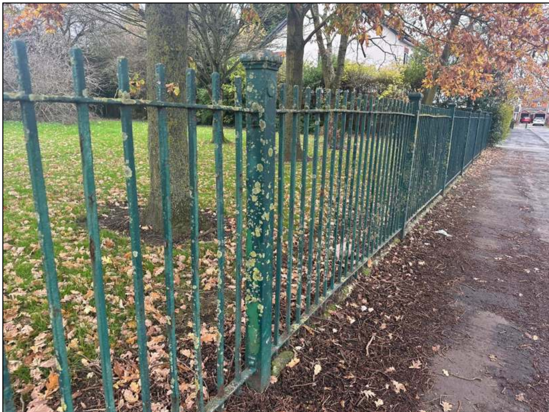
Photograph 10; The western boundary of the site comprises typical park fencing.
