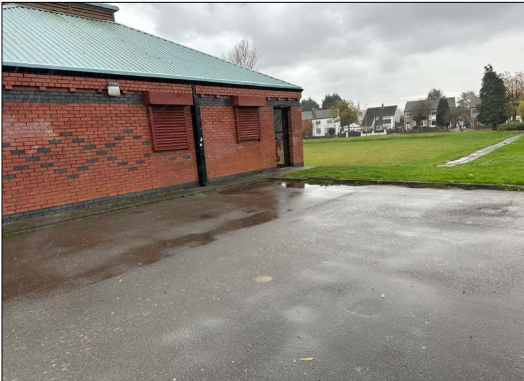
Photograph 6; A view of the pavilion building on site that is to remain. The hard standing ground currently present will be extended onto site.
