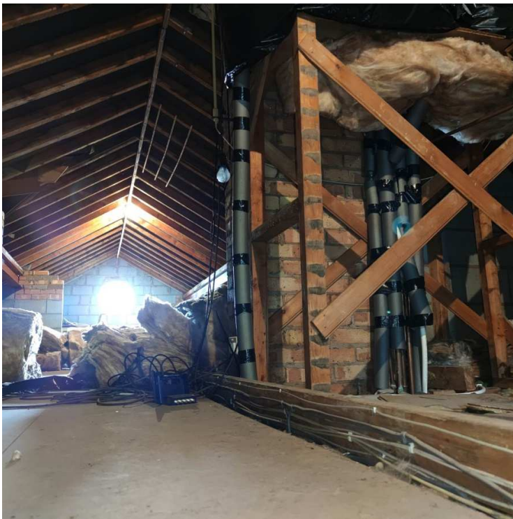
Fig 4 - Loft not currently high enough to convert
