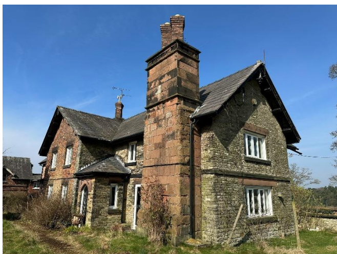
Fig. 2 – general view to rear building
