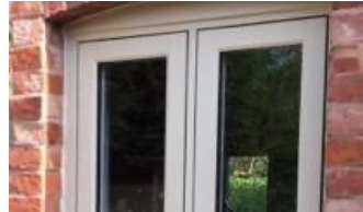
Brick double header course
