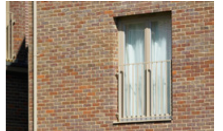
Brick double header course
