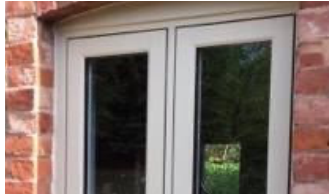
Brick double header course
